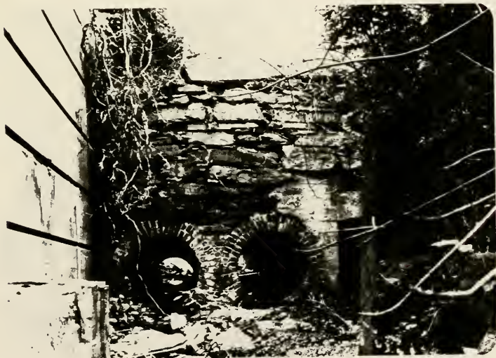
Plate 46. Dual sluice pipes in the basin below Lock 51 which appear to have fed water to the Birdsboro shop.
