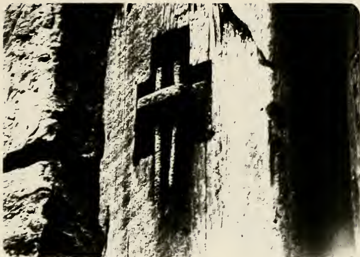
Plate 81. Beam held by iron anchor assembly outside the lower gate of Lock 53 at Laurel Hill.
