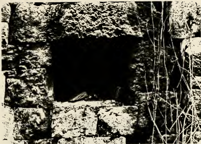
Plate 76. Detail showing one of the drainage culverts built into the lower chamber at Laurel Hill Locks.
