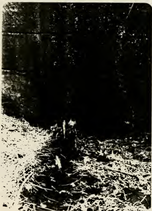
Plate 104. Remains of rotted heel post and bottom girt at Lock 57.
