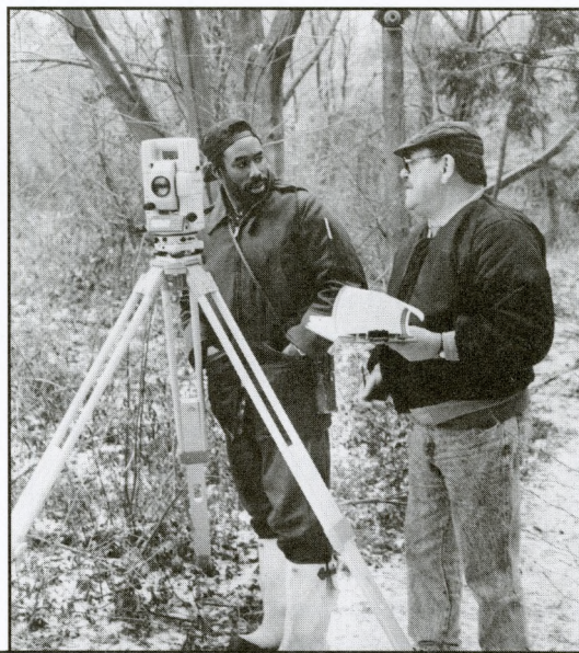
Before trenches can be dug, Survey Unit employees must layout distances for the installation of new water main and sewer pipes. Here, Ed Brown, Engineering Aide II, and Alex Faulk, Surveyor I, determine a property line near Mechanicsville Road in Northeast Philadelphia using a reflector instrument for a $1.5 million construction project.
