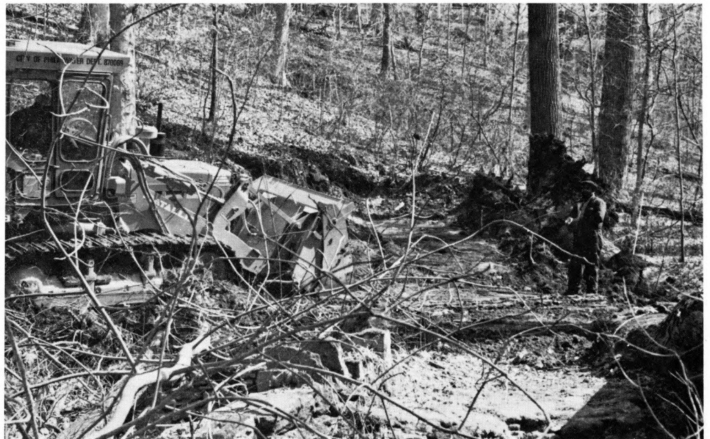
Reaching the sewer meant clearing a roadway down the steep hills of Wissahickon Park by Livezey Lane.
