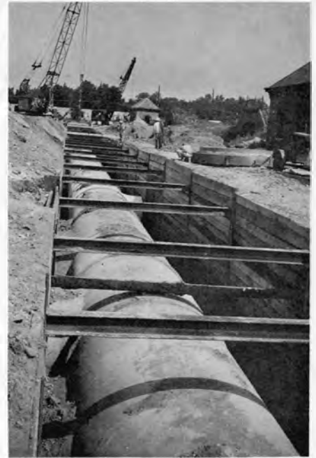
BIG CONCRETE branch main (above) will carry water to new underground storage basins at Torresdale. Water flow to basins will be measured by large Venturi tubes (above left).
