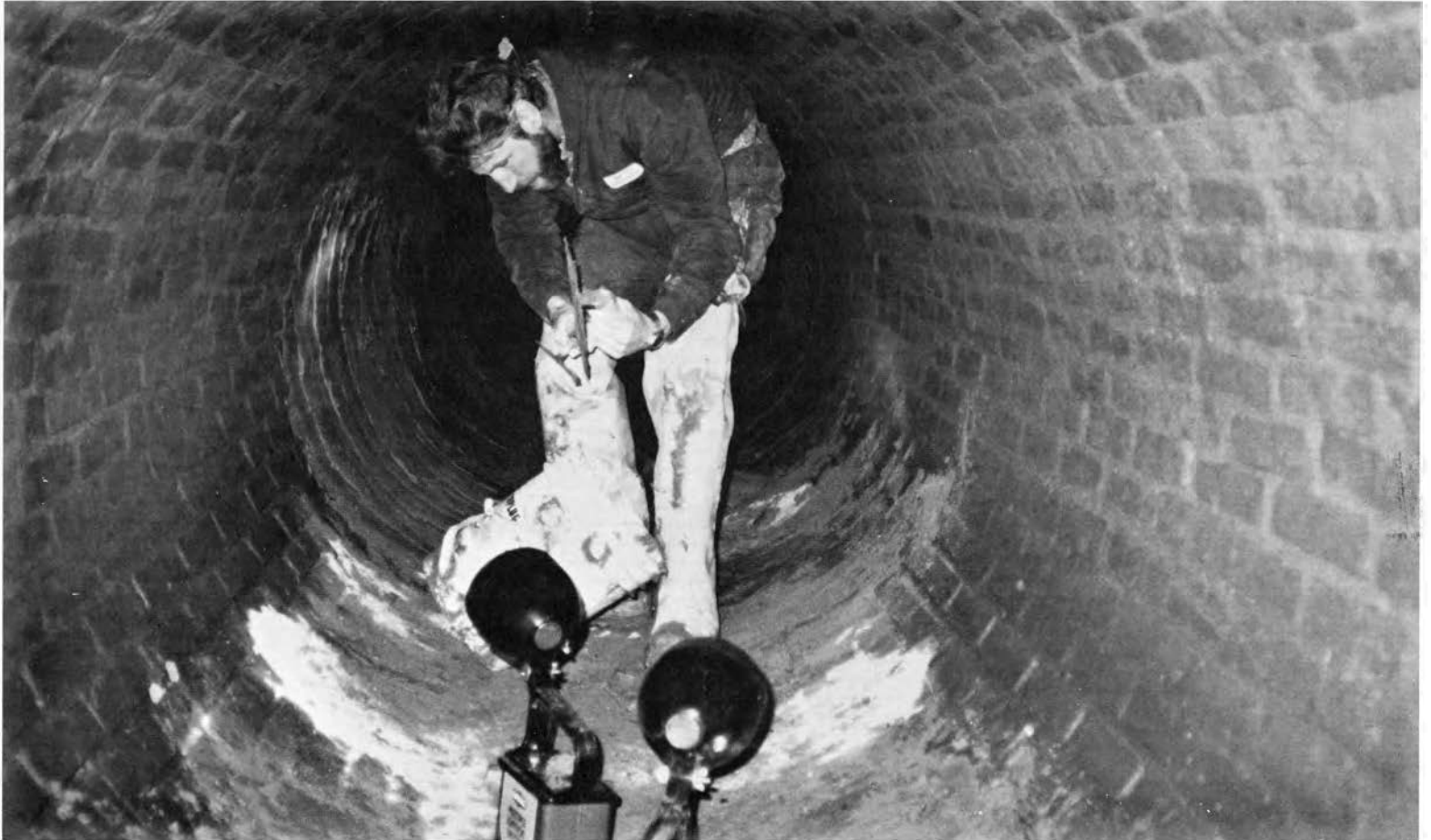
Bill Laver, SM brick mason, is repairing the invert of the brick-lined sewer with a watertight mortar mix.
