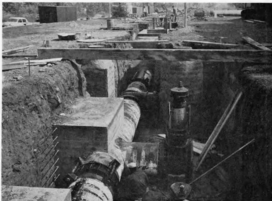
TORRESDALE FILTERED WATER Pumping Station gets new valve and pipe connections to a big feeder main that comes down from the Torresdale Treatment Plant. Job is part of station modernization.
