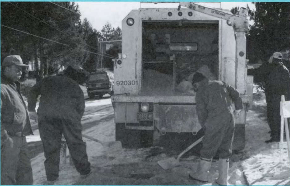
A Sewer Maintenance crew works hard on a snowy day to fix a crumbling sewer wall in Northwest Philadelphia.
