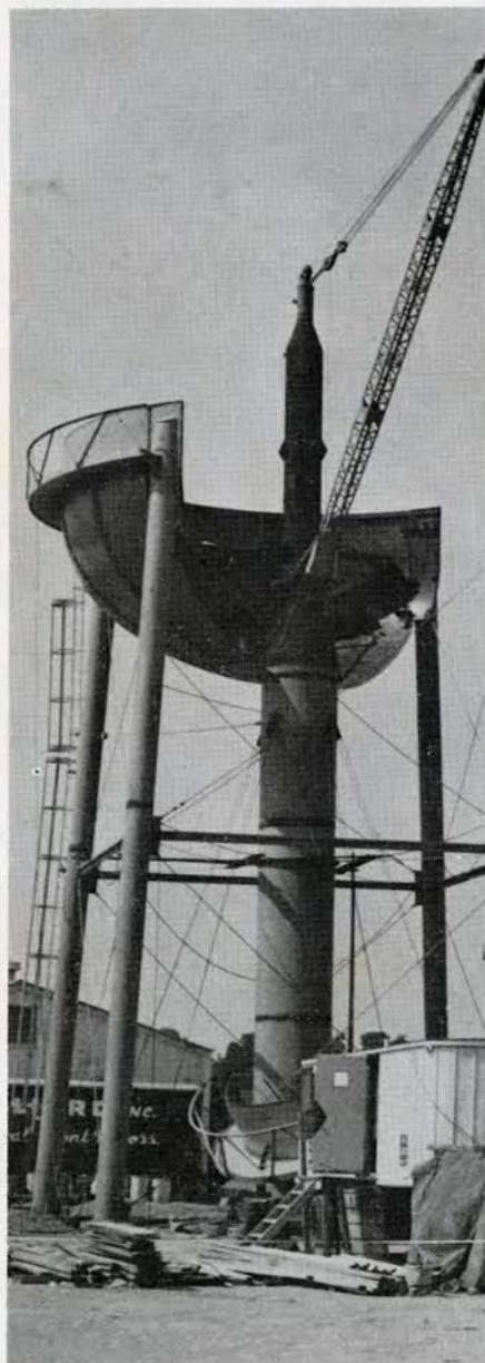
WARLIKE: Giant missile at Belmont Water Plant is harmless core of new wash water tank.
