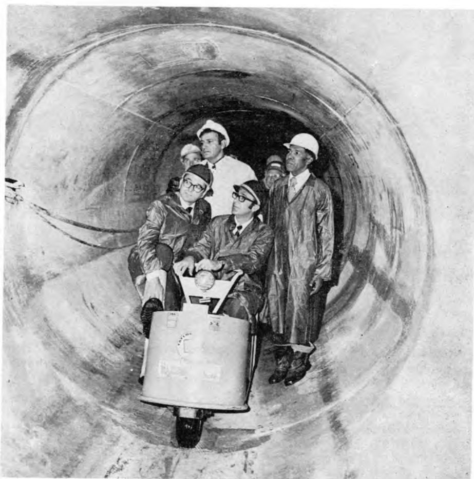
MOTOR SCOOTER is driven by Commissioner Carmen F. Guarino through a 6,000-ft. tunnel that will supply river water to the Queen Lane Plant. With him on inspection tour are Deputy Managing Director Thomas C. Piccoli (white rain coat), Deputy Commissioner Kenneth Zitomer (seated left) and Construction Chief Walter H. Clark.
