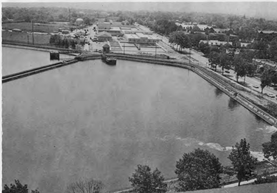
IN THIS HUGE RESERVOIR, which holds 72 million gallons, the river water is chlorinated before it flows to the new Belmont Plant (background). The water takes 22 hours to pass through the reservoir.
