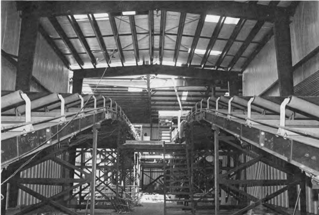
Inside of Receiving/Mixing building showing conveyor belts leading to mixing end of building
