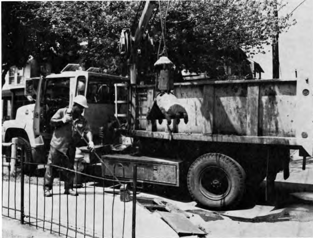
Lawrence Phillips brooms the area after the inlet has been cleaned.
