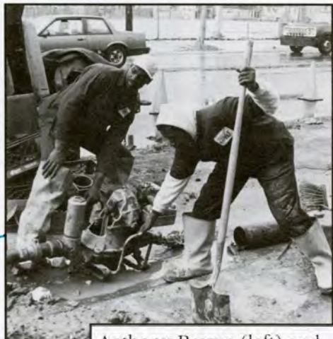
Anthony Brown (left) and Greg Pace (right) of Distribution gather up their equipment after completing an emergency repair to a hydrant line.
