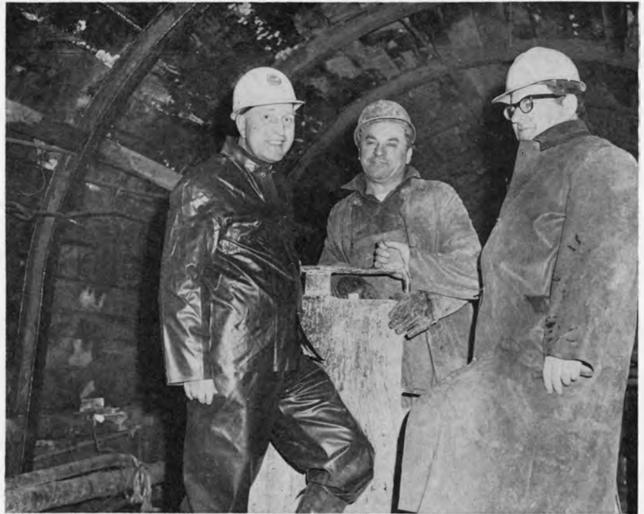
EDITOR RAY HARRIS (left) and Engineer Richard Wade (right) mount a small diesel train for a half-mile ride through the unconcreted portion of the new water tunnel. The train (photo below) moves through smoothly bored rock, cut by a rock boring machine.
