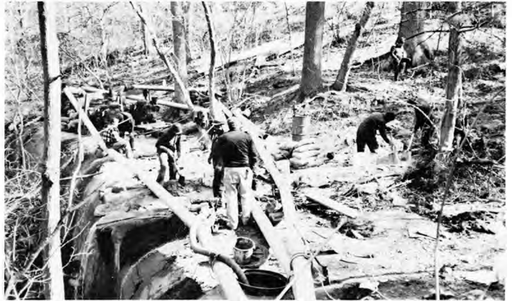
Sewer Maintenance successfully dried out the damaged section of the combined sewer by sandbagging and pumping. Pumping is continued while concrete patching material is mixed.
