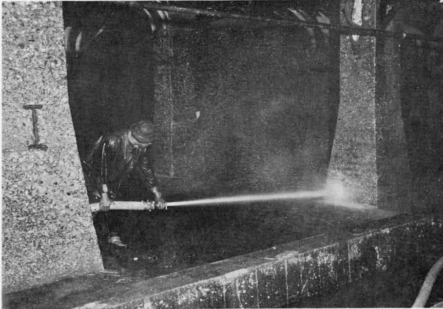
WORKMAN SEALS a crack in an underground grotto pillar by shooting a mixture of sand and cement into it under high pressure.
