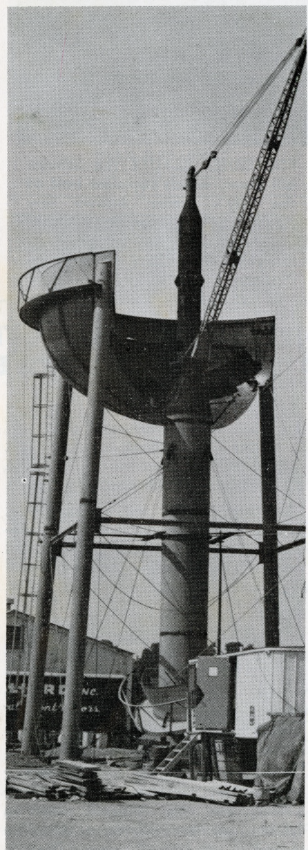
WARLIKE: Giant missile at Belmont Water Plant is harmless core of new wash water tank.
