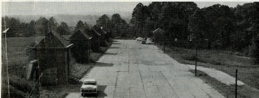
LIKE DISCIPLINED SENTINELS the small buildings at left guard the underground filter beds at the Lower Roxborough Plant. Soon to close, the plant has a capacity of 10 million gallons of water daily.
