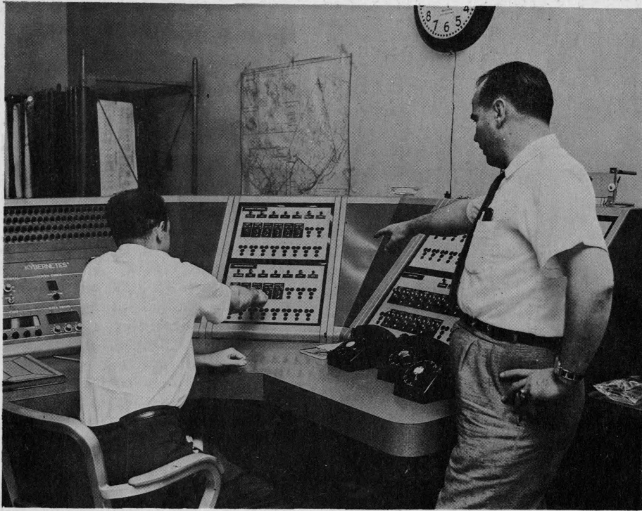
VICTOR A. PAGNOTTO (right), chief load control dispatcher, shows "trainee" Daniel J. McCusker the button to push on the panel at the new Load Control Center. Pagnotto will head one of the most unusual electronic systems in the water works field.
