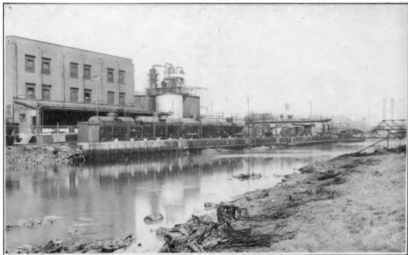
B—PRIVATELY OWNED BULKHEAD LOCATED ON NORTH BANK BETWEEN BRIDGE STREET AND MARGARET STREET. THIS BULKHEAD CAN BE INCORPORATED IN THE IMPROVED CHANNEL.
