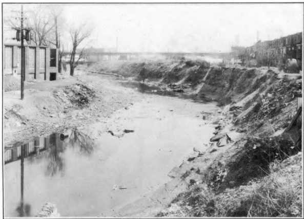
B - LOOKING DOWNSTREAM FROM LEIPER STREET TOWARDS KENSINGTON AVENUE. PROTECTION OF BANKS AT RIGHT REQUIRES HIGH WALLS OR A SECTION OF COVERED CONDUIT.
