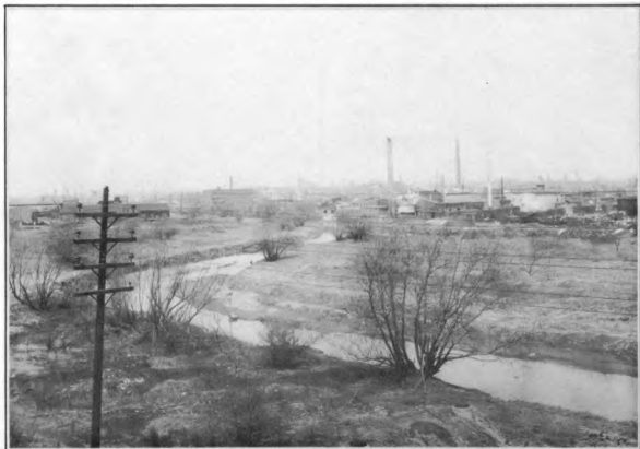
B - LOOKING UPSTREAM FROM ARAMINGO AVENUE. AN EARTH CHANNEL IS SUITABLE FOR THIS REACH
