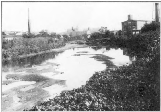
A - VIEW TAKEN NOVEMBER 10, 1932, SHOWING MILL POND FILLED WITH SEDIMENT
