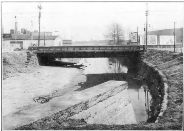
A- LOOKING DOWNSTREAM AT FRANKFORD AVENUE BRIDGE. SEDIMENT DEPOSITS RESTRICT WATERWAY OPENING
