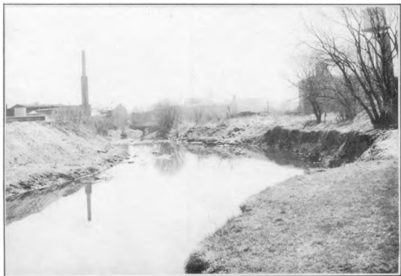
B - VIEW TAKEN APRIL 8, 1947, FOURTEEN YEARS AFTER REMOVAL OF THE DAM, SHOWING DEGRADATION OF THE STREAM BED AND BANK EROSION.
