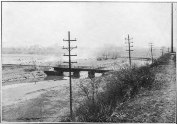
A- LOOKING DOWNSTREAM FROM ARAMINGO AVENUE. UPSTREAM END OF RECOMMENDED CUT-OFF CHANNEL TO DELAWARE RIVER WOULD BEGIN AT RIGHT OF PICTURE.
