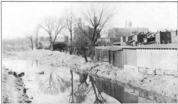
A - LOOKING UPSTREAM FROM KENSINGTON AVENUE. INADEQUATE LEVEE ALONG BANK AT RIGHT.
