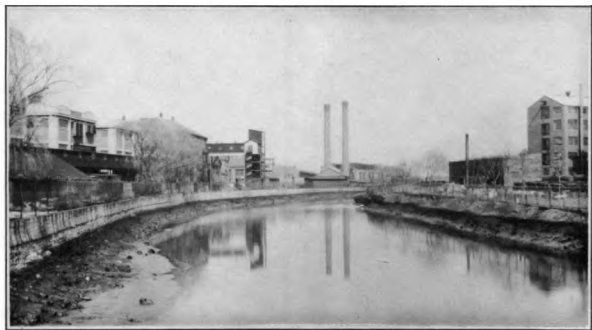
B-LOOKING DOWNSTREAM FROM BRIDGE STREET. ARSENAL WALL ON LEFT.
