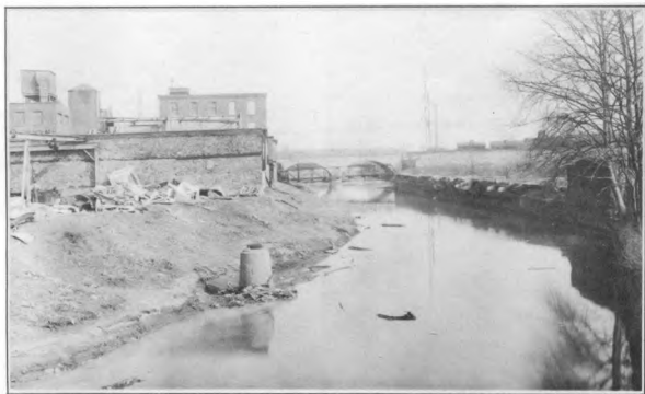
B - SAME REACH AS SHOWN ABOVE ON APRIL 8, 1947. ARCH BRIDGE IS CROSSING OF THE PENNSYLVANIA RAILROAD. STEEL TRUSS FOOTBRIDGE HAS BEEN ABANDONED.
