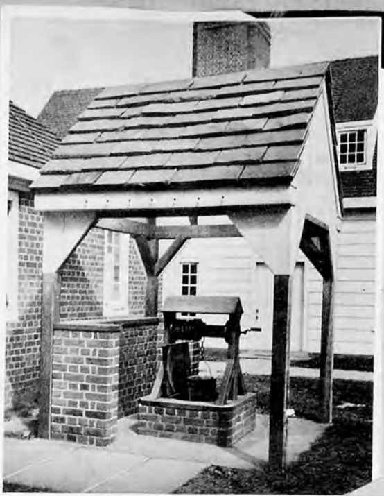
6—The well, strategically placed just outside the kitchen door.
