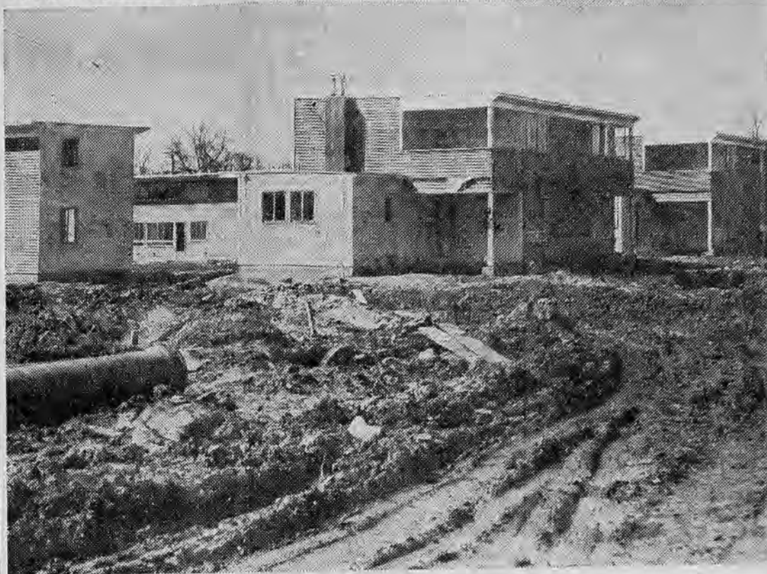
Part of the Pennypack Woods defense housing development which private builders say violates city building code. The buildings, of frame, are called "fire traps. The structure in middle is for four families
