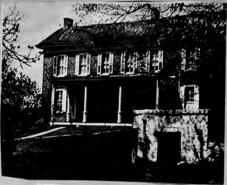
Washington's Headquarters in Newtown, after the Battle of Trenton, were in a brownstone house at Sycamore Street and Washington Avenue. The present house, the third on the site, is believed built of stone of the Headquarters House and on the original foundation.
