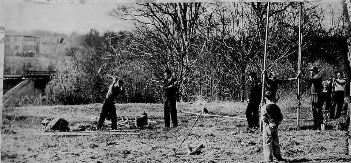
Erection of the 32-foot trapeze rigging presented some problems. Greatest was uneven ground; another was the replacement of old rope, as the equipment had been in storage for the last five years while the boys were in service. Supports are of steel tubing made up in sections for dismantling.
