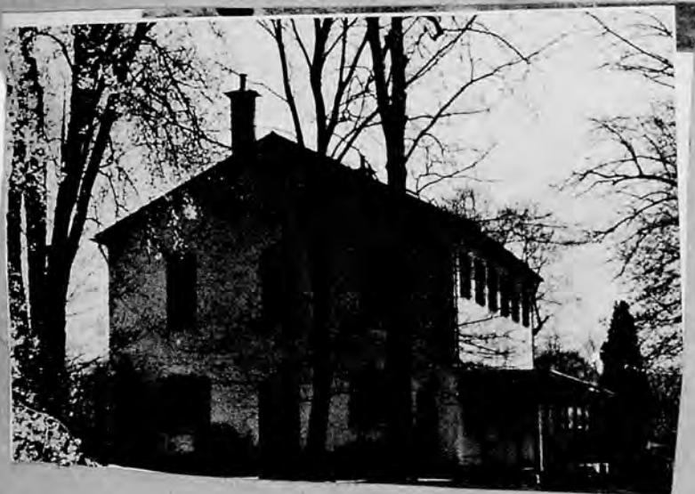
The history of Newtown Meeting House, a booklet on which has been published by the "Newtown Enterprise," is particularly interesting. The first ground purchased by Newtown Preparative Meeting of Friends upon which the meeting house was erected was made in 1818.
