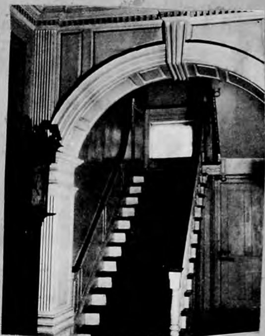
In 1764, Amos Strickland built the house now known as the Brick Hotel. The moulding and the detail of the staircase are of the finest type of woodwork and carving. The original doors are paneled on both sides.
