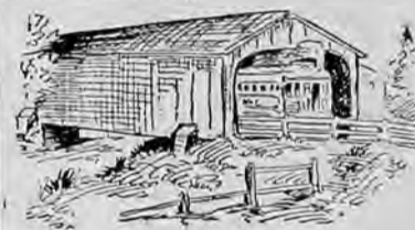
OLD "DUMMY" BRIDGE Over Frankford Creek.
