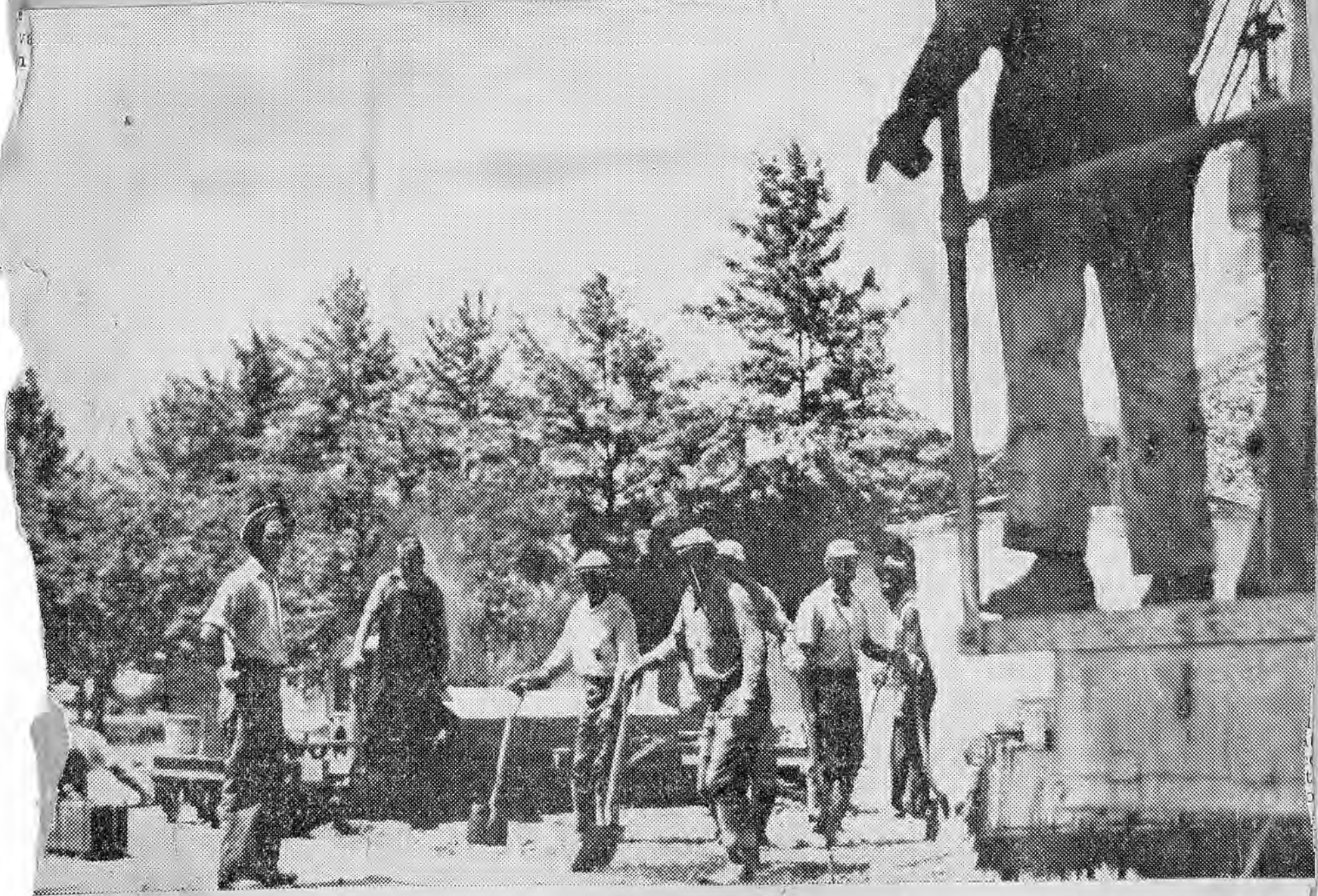
NG the concrete is also done by the mixer, but workmen spread it with their shovels and the
