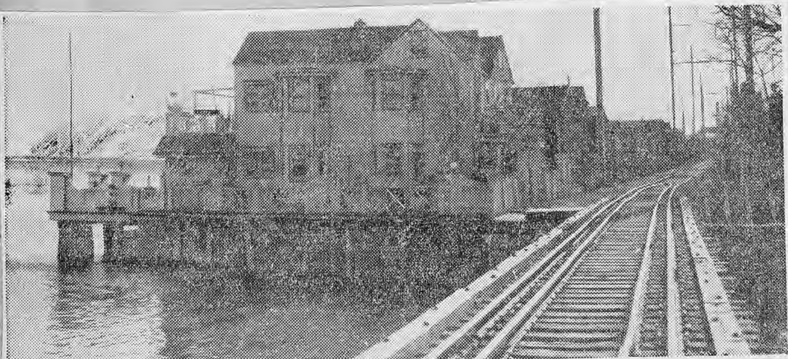
REMINISCENT of the days when the upper Delaware was the boating and fishing center of Philadelphia, are these homes along Delaware ave., at the foot of Devereaux st. Despite pollution of the stream by dyeing, chemical plants (fishing ended 20 years ago), boating enthusiasts still maintain flourishing clubs in the vicinity. Best known are the Wissinoming Yacht Club (119 members, 54 craft); Quaker City (106 members); Red Dragon Canoe Club. Regattas are held here annually. Old Wissinoming names: Castor, Hanson, Campbell, Mace.
