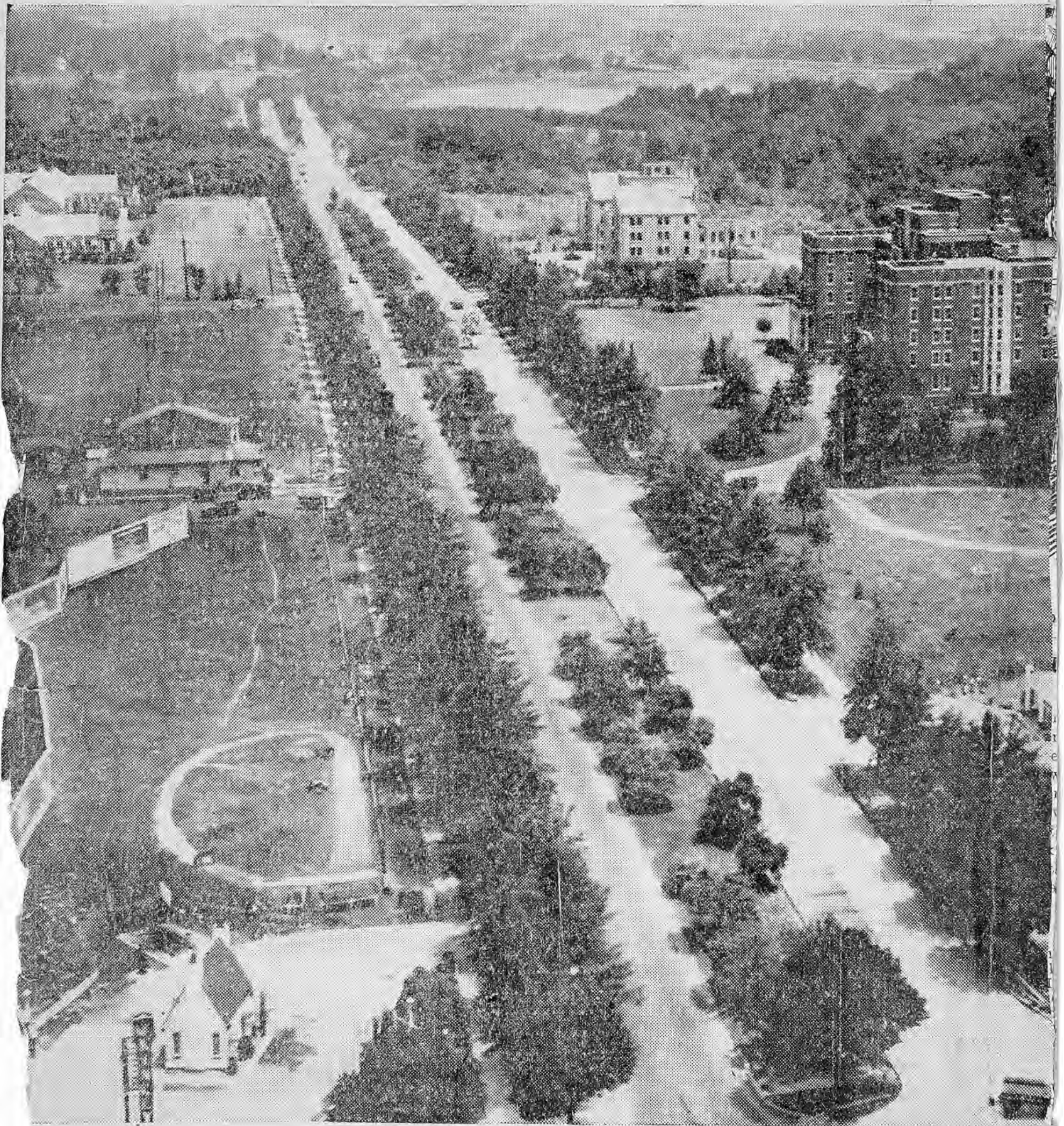
VIEW of the Roosevelt Boulevard project made by Gus Pasquarella from a Boulevard Air e. The Shriners Hospital is at left and the Evangelical and Baptist Homes are at right
