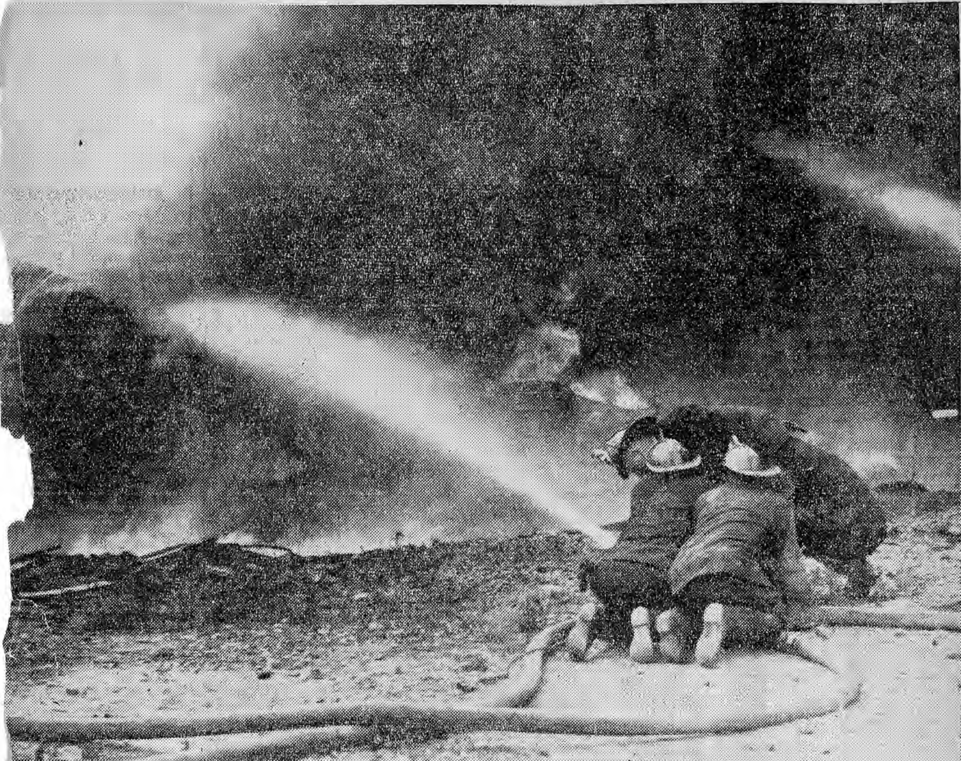
Two firemen handle one hose line in an effort to beat out fire in the foundations of the export shed at the Tiona Petroleum Company plant, Tulip and Wyngate sts., where a four-alarm blaze destroyed thousands
