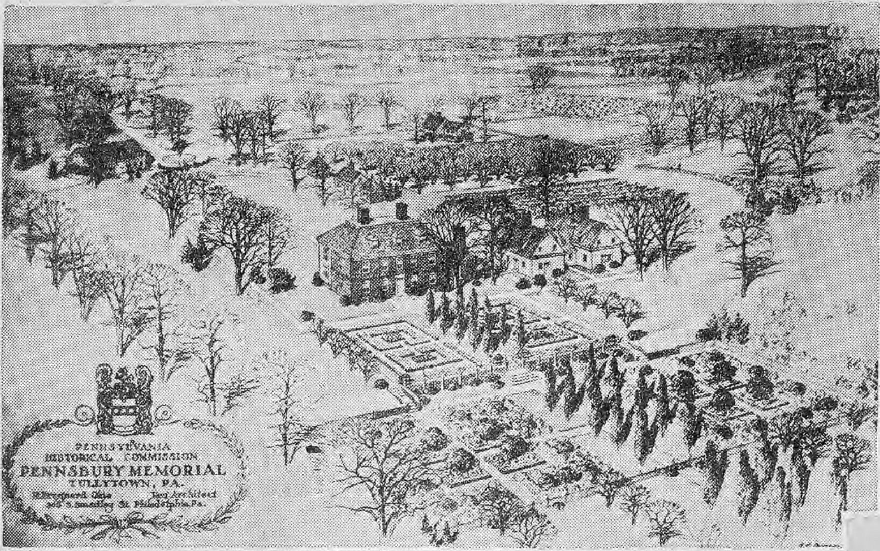
For this plan of a reconstructed Pennsbury Manor, Penn's mansion house when he was Lord Proprietary of Pennsylvania, R. Brognard Okie, local architect, studied excavations, history and old records
