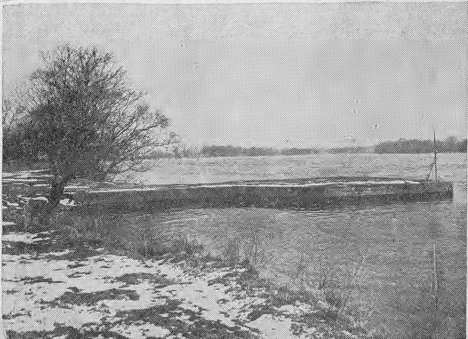
Governor Penn traveled to Philadelphia and back in a six-oared barge when "Pennepacka and Poquessing bridges" were not passable. This pier juts into Delaware at same point as original landing place.
