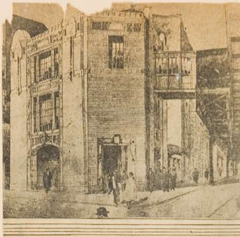
Sketch of one of the Frankford elevated stations, which shows that these new stations are located back of the building lines and connected to the elevated with a bridge. Both its architecture and its physical usefulness show that these buildings have been carefully designed and that they will be a credit to the city.
