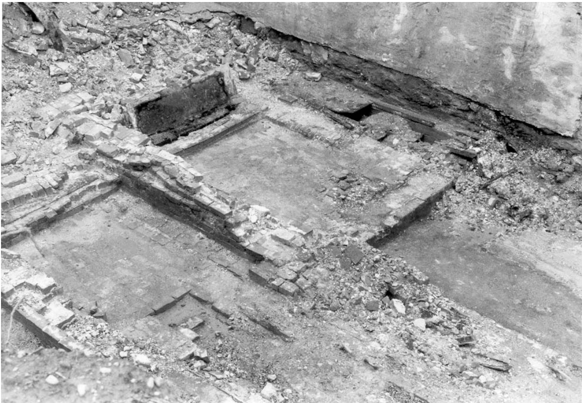
A-27. Drainage and storage features under concrete basement floor, 529 Market Street, view east-northeast.
