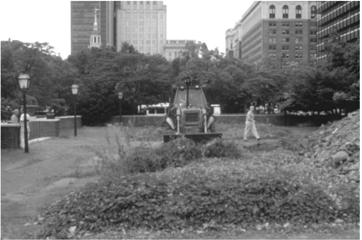
Figure 10. Backhoe beginning to remove landscape on Block 2.
