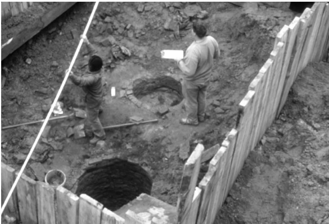
Figure 17. Shoring box around Features C and D.
