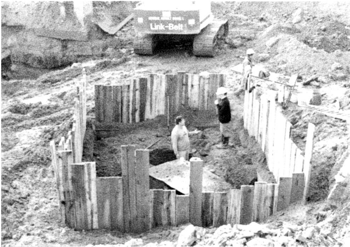
A-7. Wooden plank-and-beam shoring box around Features C and D during Phase III, view south-southeast.
