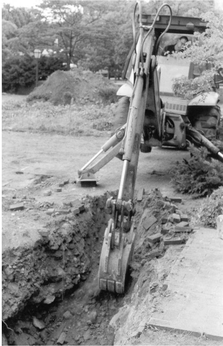
A-2. Initial backhoe (Case 580) used to excavate trenches.
