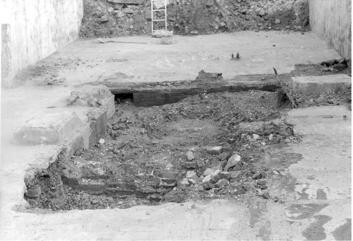
A-24. Probable sump pit set into concrete basement floor of 529 Market Street, view north-northeast.
