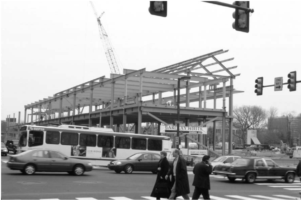
Figure 33. Independence Visitor Center under construction, November 2001.
