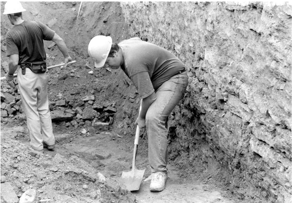
A-4. Manual cleaning of basement floors.
