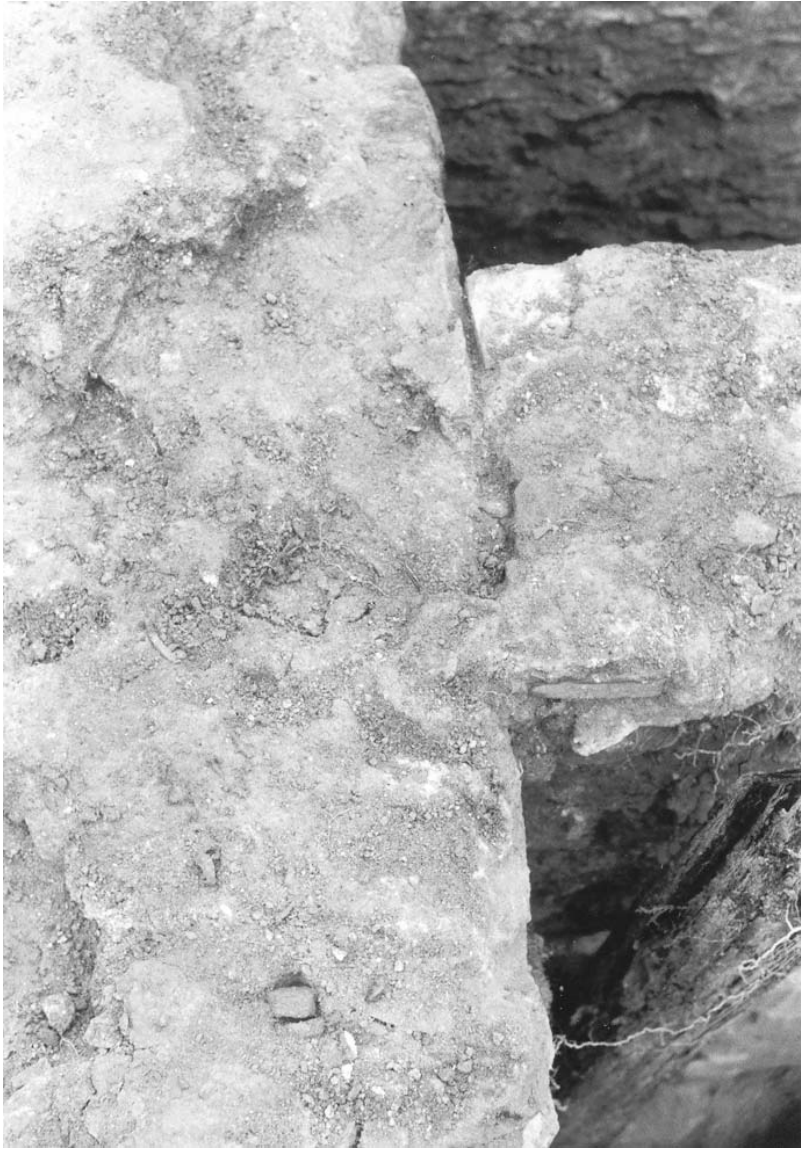
A-20. Butt joint at southwest corner of 528 Commerce Street, view west-northwest.
