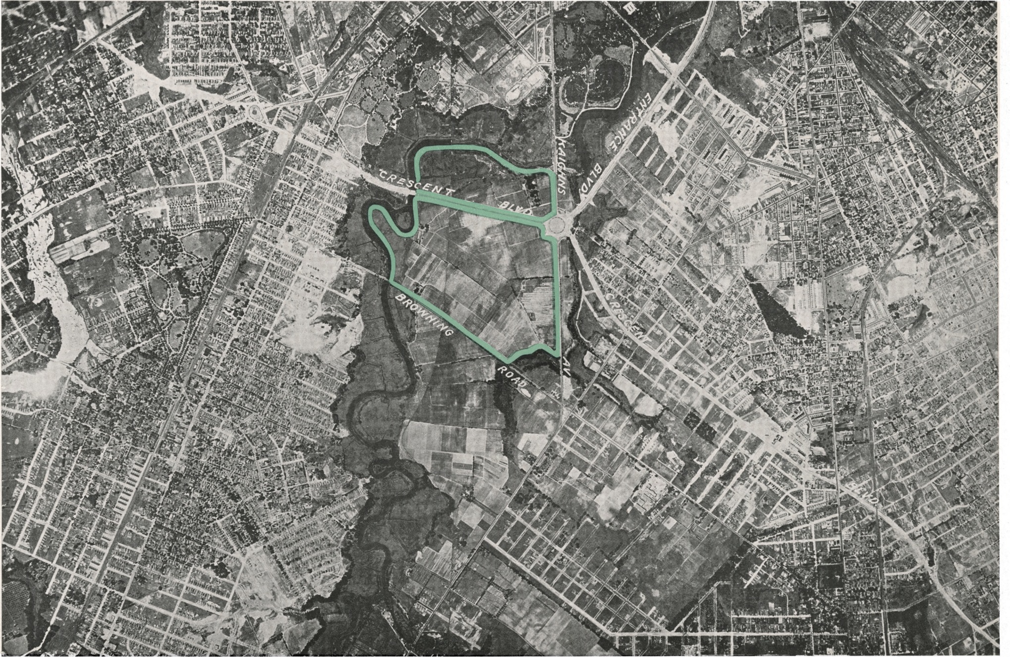
SITE OF PROPOSED "CENTRAL AIRPORT," NEAR CAMDEN, N. J. AERIAL VIEW—VERTICAL
