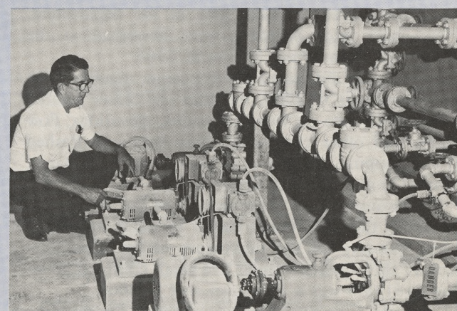
For Taste and Odor Control: West Philadelphians were due to receive even better water in mid-1967 as the result of a new ammonia feed system, almost completed at the Belmont Water Treatment Plant. By treating the water with carefully controlled doses of ammonia, the system will eliminate some tastes and odors. Photos: System control panel at left; ammonia pumps and piping above.
