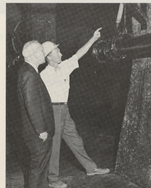
Underground Reservoir. As part of a plan to increase underground storage for purified water at all the water treatment plants, three basins began to take shape at the Belmont Plant. Piping (above) will carry off the rain water from the roof, protecting the stored water.
