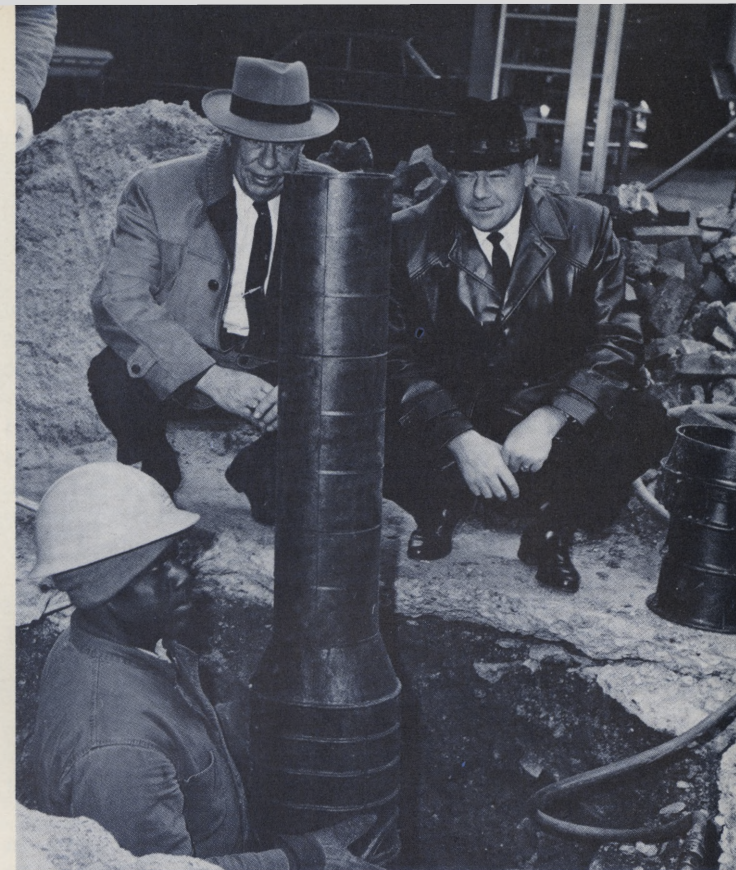
For Big Savings: A new type of valve box, made of plastic, was used by the Water Department for the first time. Saving the department over $100,000 a year, the valve box weighs only two pounds, eliminates injuries, and is adjustable in length.
