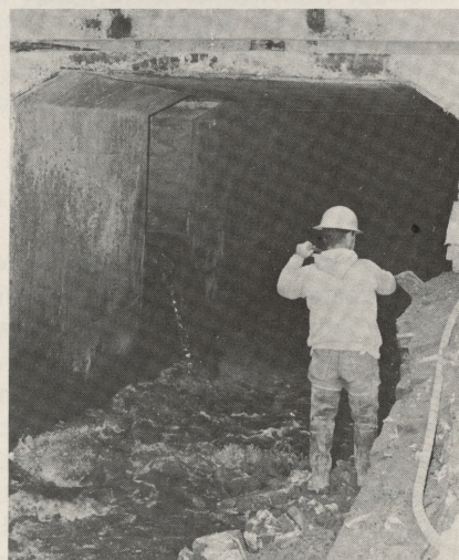
Gunner's Run Sewer: Built partly in open cut and partly in tunnel, the $2.1 million sewer was almost finished. In photo, concrete section of new line and some 70-year old bricks of old sewer.
