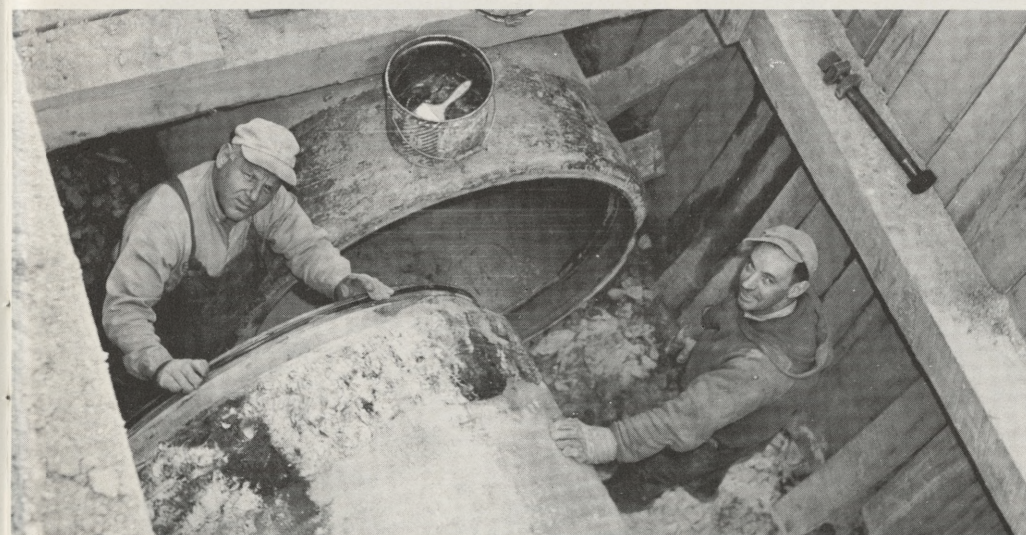
For Water Supply: More than 33 miles of new water mains were constructed in 1966 to serve new homes and industries as well as to replace old mains. Some of the biggest pipelines, ranging up to four feet in diameter (photos), were laid to supply new underground basins at the Belmont Water Treatment Plant.
