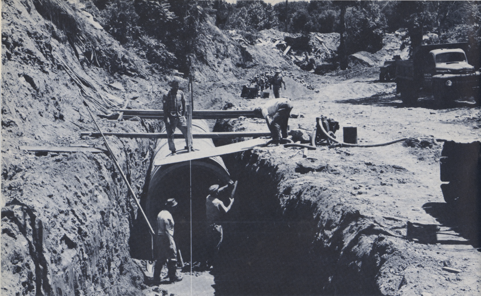
Drainage: A large sewer is laid in a Northeast Philadelphia drainage right-of-way to assure better storm water run-off to neighboring streams. Water Department crews inspected 148 drainage right-of-way locations in 1966 and cleaned over half of them.
