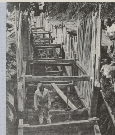
Toward Improved Sanitation: About 2.3 miles of sewers were built in 1966 to provide City sewer service for some homes for the first time. Above, workmen place wooden sheathing and shoring for a sewer in Rex Avenue, while below a pipeline is run beneath the Schuylkill Canal to carry wastewater from Roxborough-Manayunk to an interceptor.
