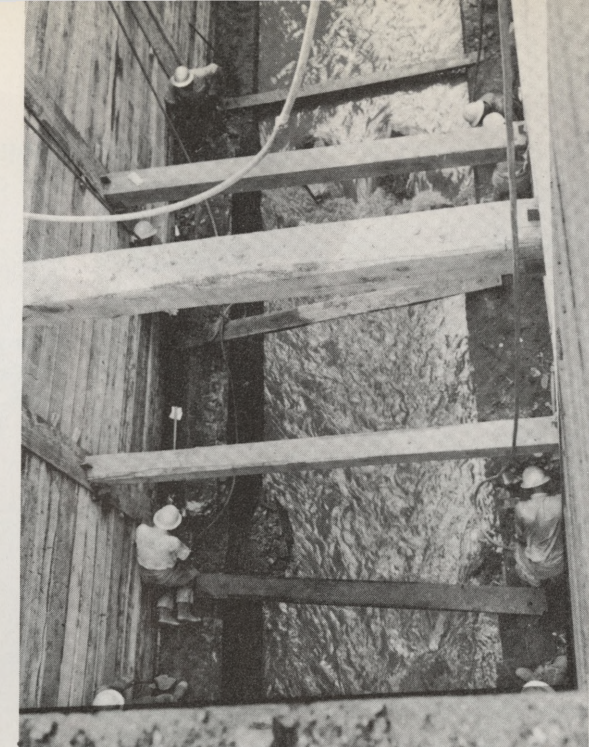
Sewer Replacement: Work started on replacement of the deteriorating Gunner's Run Sewer, which picks up storm and sanitary flow from large areas in North Philadelphia. In all, about nine miles of old sewers were replaced throughout the city.
