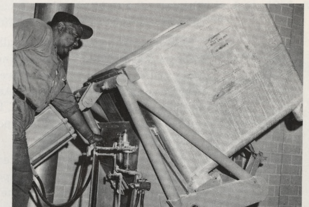
Hexametaphosphate: Automatic equipment unloads hexametaphosphate into storage bins. This chemical helps to control corrosion of mains in the distribution system, thus reducing water discoloration.
