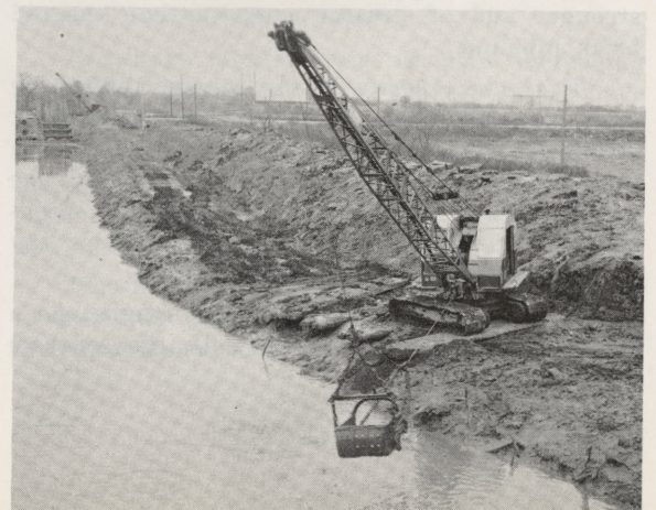
Storm Flood Control: To carry off storm flow, the long Main Relief Sewer was further extended to 16th Street and Allegheny Avenue in North Philadelphia while Mingo Creek was deepened and widened in Eastwick. The creek was being transformed into a mile long surge basin to support a new storm water pumping station.
