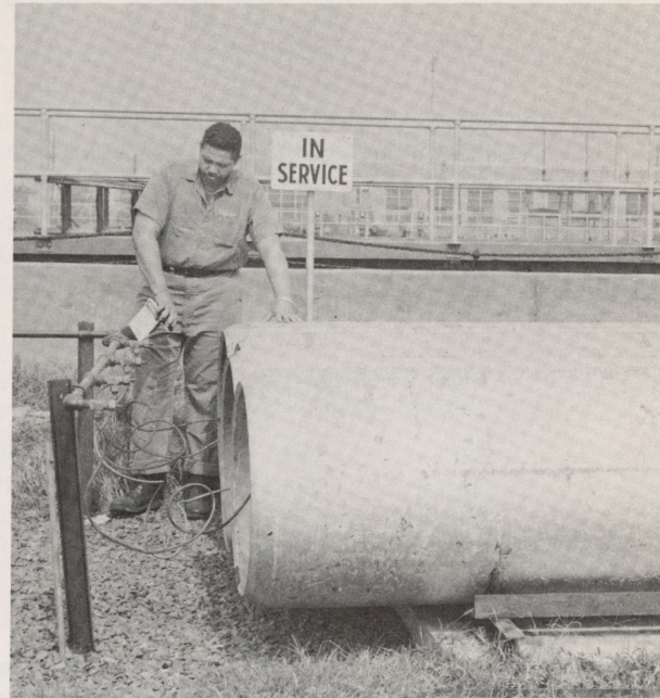
For Stream Protection: At the Southwest Plant chlorination began of the liquid effluent that enters the river after wastewater treatment. Tanks in photo supply chlorine to chlorination equipment in the small building.
