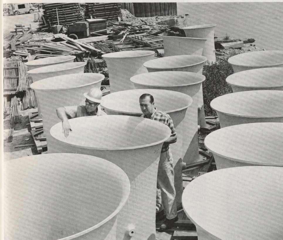
For Capacity: To meet the needs of half the City of Philadelphia, 16 huge flow nozzles were readied for placement beneath the new Torresdale intake. The specially shaped nozzles will permit the use of automatic equipment to measure water volume.
