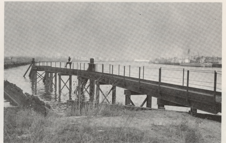
Barging of Sludge to Sea: A new loading dock takes shape on the Schuylkill River. The dock will serve barges that will haul digested sludge to sea from the Southwest Water Pollution Control Plant. Digested sludge is the innocuous residue of wastewater treatment.
