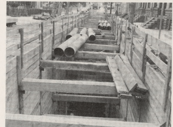
Storm Flood Control: To carry off storm flow, the long Main Relief Sewer was further extended to 16th Street and Allegheny Avenue in North Philadelphia while Mingo Creek was deepened and widened in Eastwick. The creek was being transformed into a mile long surge basin to support a new storm water pumping station.
