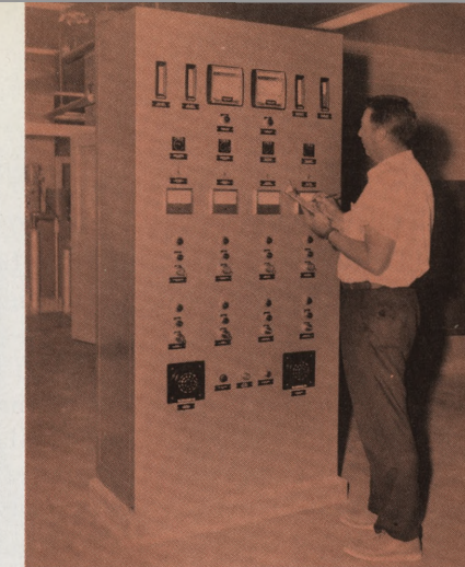
An Automated Plant: Monitored and controlled by automatic or semi-automatic devices, the operations at the new Belmont Plant will be much more efficient than were those in the plant it replaced. Panels at left and center record and regulate chemical feed; panel at right controls filters.
