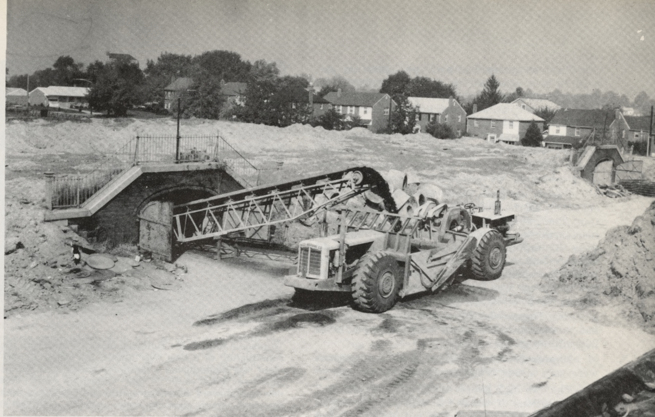
Future Water Storage: Sand pours from one of the abandoned filter beds at the former Upper Roxborough Water Plant as work starts on the conversion of eight beds into an underground reservoir for purified water. More than 34,000 cubic yards of sand and gravel were removed.
