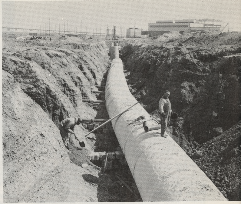
Sewers for New Development: More sewers were built in 1965 to service new homes and industries than for any other purpose. Photos show big storm water pipelines taking shape in the Northeast (left) and Eastwick (right), two of the city's most important new areas. Many sanitary pipelines were also laid.
