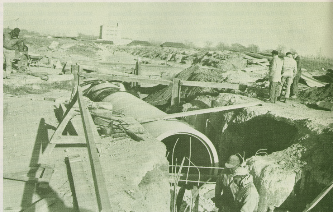
Water Storage: Conversion of old slow sand filters at the Torresdale Water Plant into underground reservoirs for filtered water continued. The $4.2 million job will provide additional storage for 143 million gallons.
