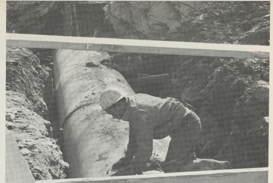
Schuylkill East Bank: A 3.5 mile intercepting sewer along East River Drive was nearly finished. Workmen place a tributary connection above.
