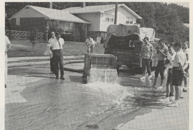
Sewer Inlet Study: To improve the future design efficiency of sewer inlets, the Research and Development Unit made various field studies. Inlet slope, grate size, other factors, were noted.
