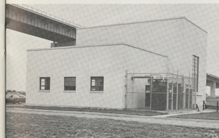
Mingo Creek Station: A new $965,000 station stood ready to pump storm water from Mingo Creek into the Schuylkill River. Still to be tested at year's end, the new station will be able to pump 123,000 gallons of storm water per minute initially.
