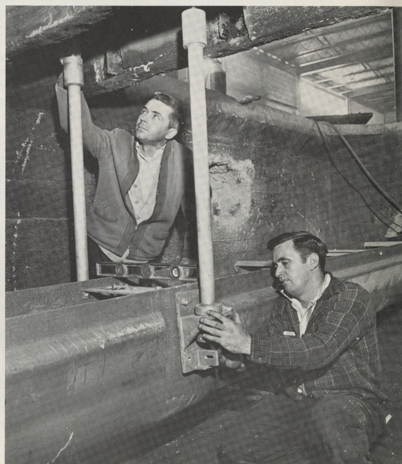
Belmont Plant: Construction of the north wing of the new filter building was well advanced by the end of 1964. Typical filter bottom (right) will go into 12 new rapid sand filter beds, each capable of processing three million gallons of water daily.
