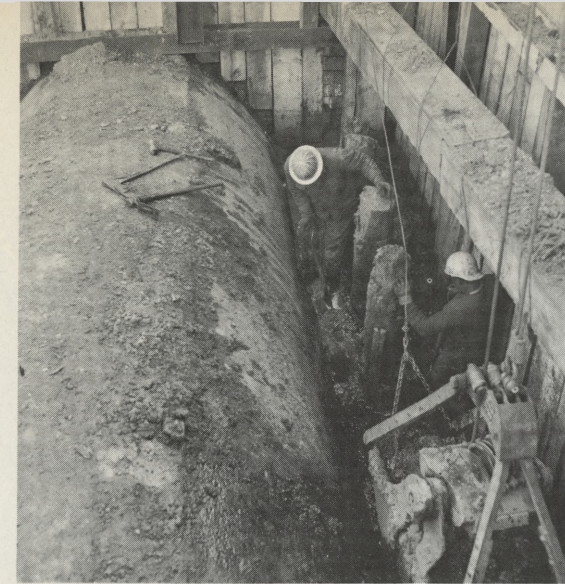
Schuylkill West Bank: Workmen remove earth for construction of a new intercepting chamber. Latter will form part of a long intercepting sewer, extended for a half-mile in 1964.
