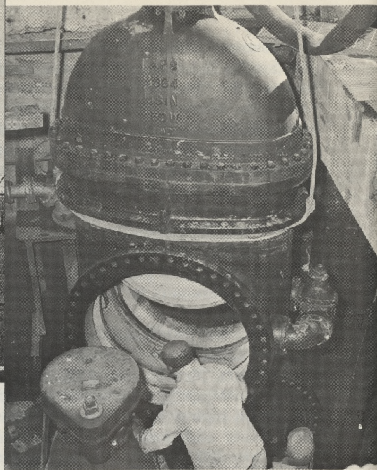
Lardner's Point: Landscaping and new valves were final touches in extensive improvements made in the past decade at Philadelphia's biggest filtered water pumping station. Valves went into huge chambers serving distribution pipelines.
