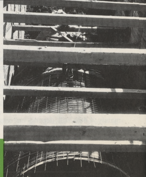
Mill Creek Sewer: For better storm flood control, the old brick sewer was replaced in Farragut Street for 150 feet with a new reinforced concrete line (above). Section of new sewer with reinforcing, right.
