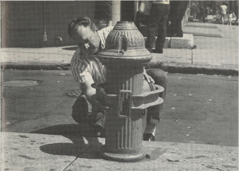
Fire Hydrant Protection: To prevent hundreds of illegal summer-time openings of fire hydrants, the Water Department successfully developed a new type of steel locking device. It was planned to put such devices on 1,500 of the most abused hydrants in 1965.
