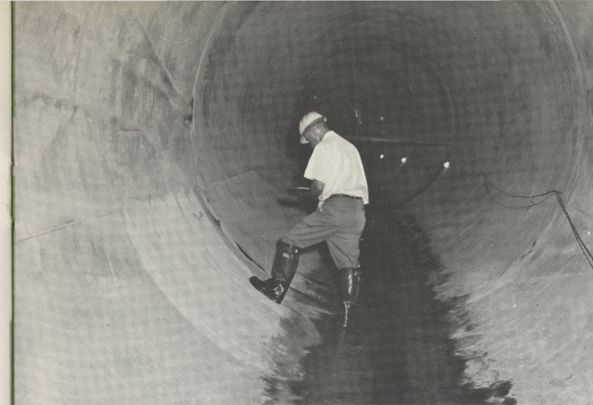
Storm Relief for South Philadelphia: The new $3 million Passyunk Avenue Relief Sewer was nearly completed. The sewer will pour 209,000 gallons of storm water per minute into the Schuylkill River.
