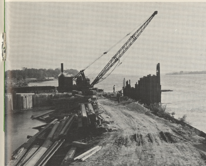
New Torresdale Intake: Work began on new push-button facilities for funneling Delaware River water to the Torresdale Water Treatment Plant. The $2.1 million job will include sluice gates, rakes, screens, valves, and chlorinators, all automatically controlled.
