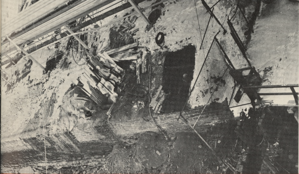
For Flood Relief: In South Philadelphia a big storm relief sewer moved along Passyunk Avenue to the Schuylkill River. Built half in open cut and half in tunnel, the sewer will carry up to 209,000 gallons of storm water per minute. Tunnel, above, lined with wooden sheathing, emerges at river below. Vertical shaft to tunnel at right.
