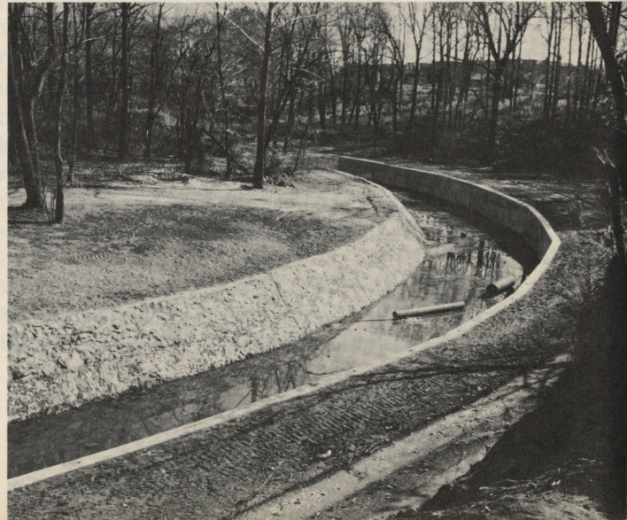
For Drainage: To carry away storm run-off more efficiently, a concrete walled channel with stone bed was built for Sandy Run in Pennypack Creek Park. Improvements were also made to stream channels in other parts of the city.
