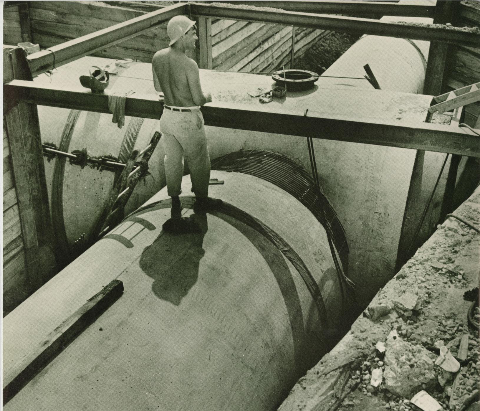
Water for all: Water continued to be big business in Philadelphia in 1963 as 326 million gallons were consumed daily. To assure a plentiful future supply, one of the biggest pipe crosses (above) in the Eastern United States was laid near the Torresdale Water Treatment Plant. The piping will supply new storage basins.
