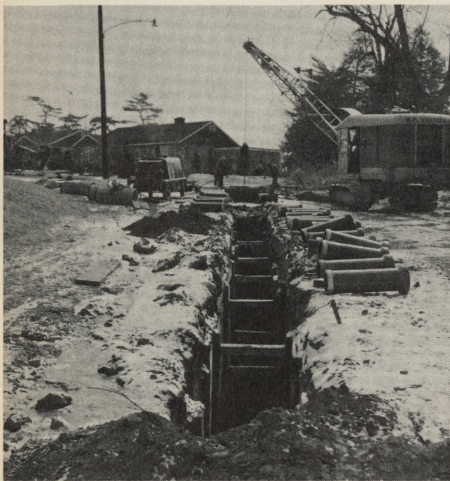
For Sanitation: 3.7 miles of sanitary and small storm sewers were laid to service existing homes. Above, sewer goes in at Bickley St.
