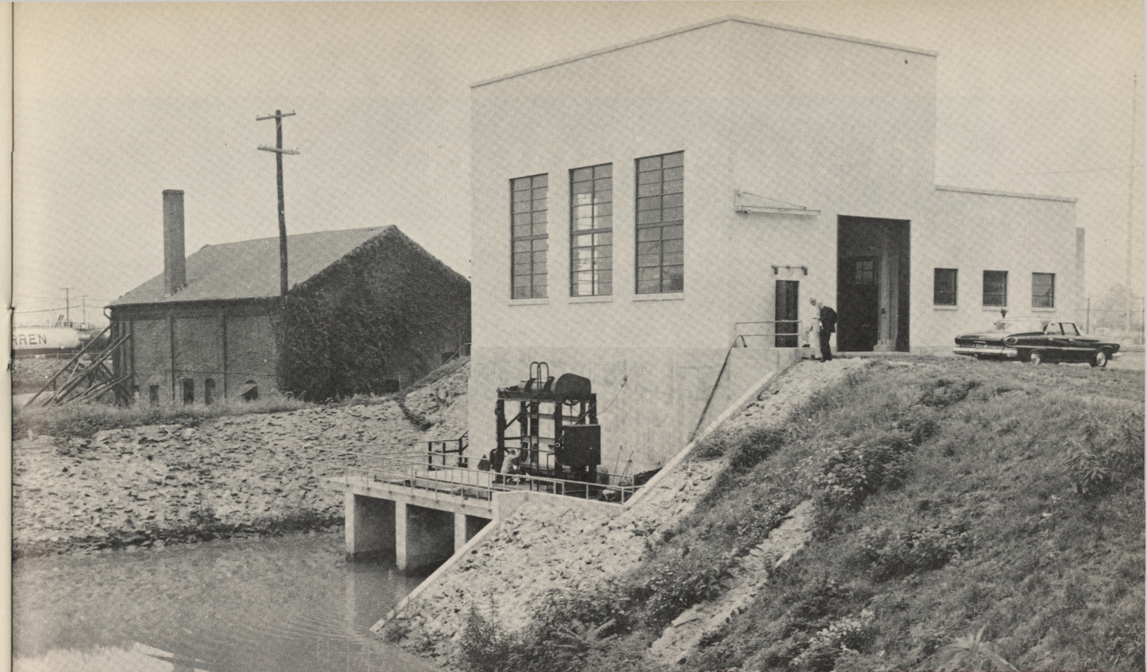
Mingo Creek Station: Nearly completed was the new storm water pumping station at Mingo Creek just north of the Penrose Avenue Bridge. The $965,000 station, which will lift storm water from Mingo Creek into the Schuylkill River, will serve Eastwick and the International Airport. Old station in background will be torn down.
