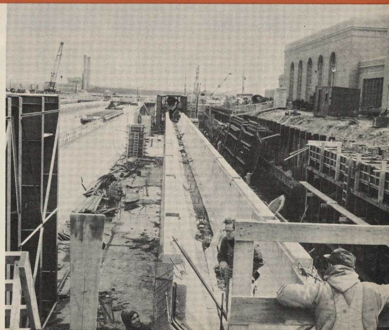
Nearing Completion: A new aeration tank takes form as part of a $5.3 million expansion at Northeast Works. Built of reinforced concrete, the aeration tank is 412 feet long, 95 feet wide, and 17 feet deep.
