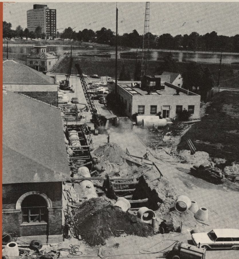
New Water Line: Crane lowers section of big conduit into place at the Belmont Water Treatment Plant. The reinforced concrete line, measuring 5½ feet in diameter, will carry river water from the pre-sedimentation basins in background to new treatment facilities.
