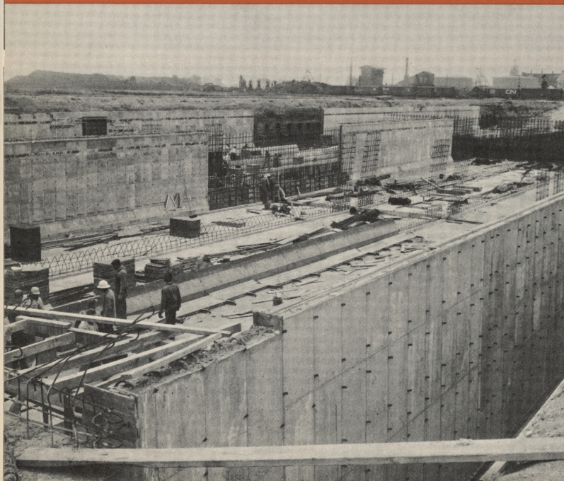
Plant Expansion: One of four final settling tanks under construction at the Northeast Sewage Works will raise that plant's daily treatment capacity from 125 million gallons to 175 million. Each tank will hold 1.4 million gallons.
