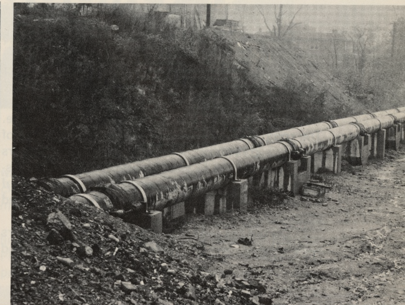
Engineering Feat: Twin water mains on piers in Silverwood Street solved a difficult problem of terrain and soil. The concrete piers, 20 feet in height, were sunk deep into the soil, and both mains and piers were covered up to grade.
