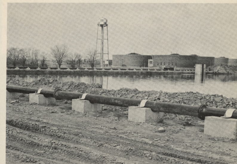
Southwest Sewage Works: New piping carried sewage sludge to a partially finished lagoon above. With sewage flow to the plant increasing, the existing lagoons at the Southwest Works were full.
