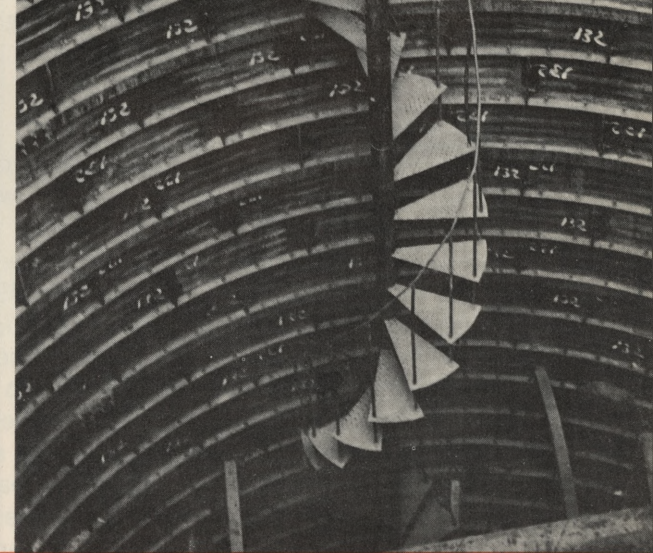
For Flood Relief: In South Philadelphia a big storm relief sewer moved along Passyunk Avenue to the Schuylkill River. Built half in open cut and half in tunnel, the sewer will carry up to 209,000 gallons of storm water per minute. Tunnel, above, lined with wooden sheathing, emerges at river below. Vertical shaft to tunnel at right.
