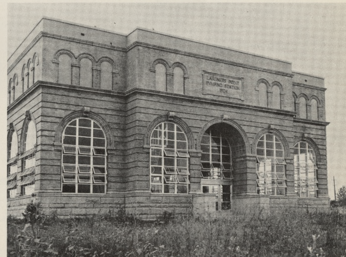
Lardner's Point: Final phase in $3.4 million modernization of this water pumping station was installation of aluminum-frame windows and doors, pointing and cleaning of exterior, and lowering of roof. Landscaping was still to come.
