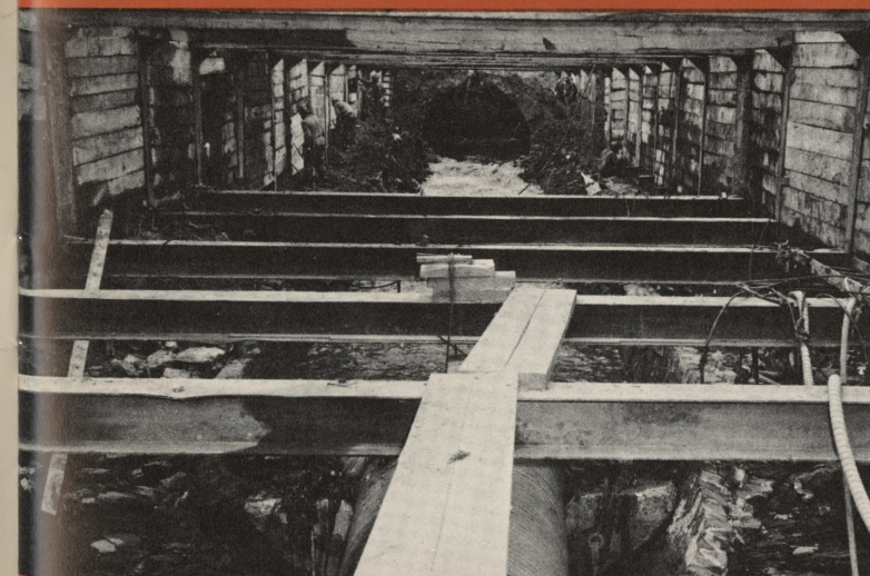
For Flood Control: Two sewers to control storm flooding were among Accelerated Public Works Projects. The old Mill Creek Sewer in West Philadelphia (above) was being replaced, while a new sewer was being built in Passyunk Avenue in South Philadelphia (right).
