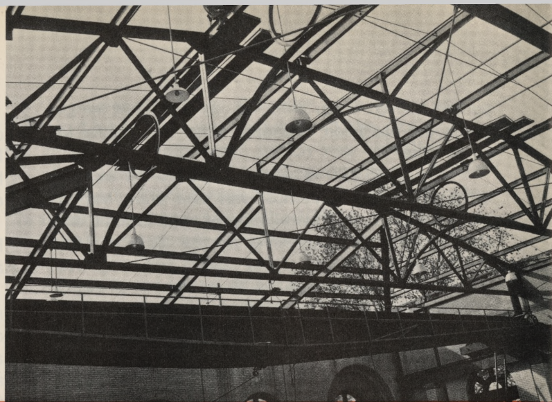
Fairhill: A new roof goes on the Fairhill High Pressure Pumping Station as part of nearly completed modernization. New pumps were installed the year before.
