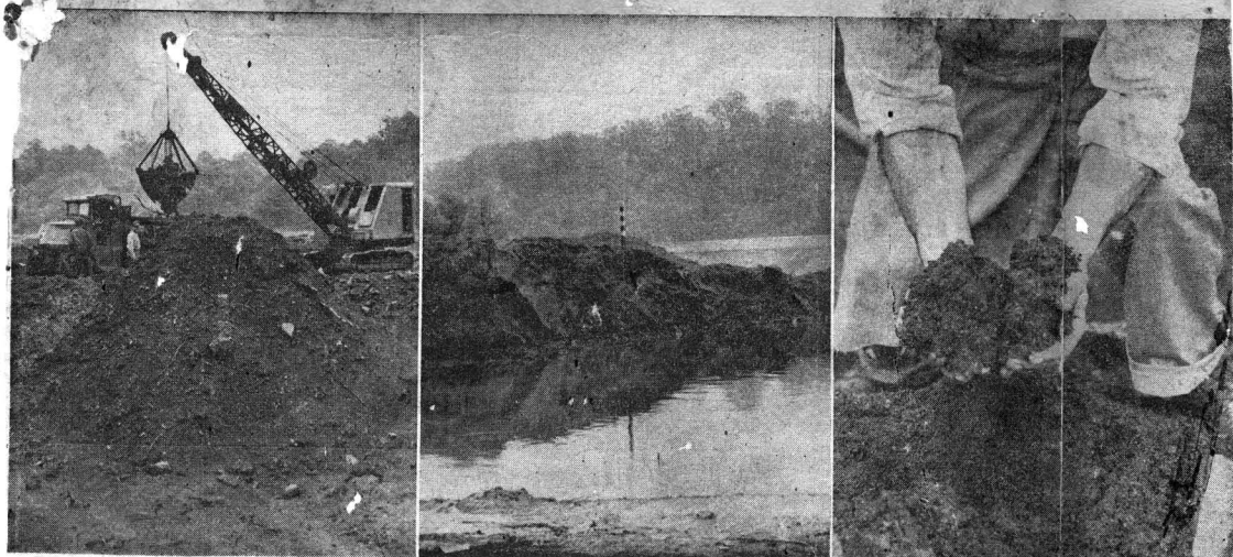
EVEN POWER DREDGES MAKE LITTLE IMPRESSION ON MOUNTAINS OF SILT LINING THE SCHUYLKILL Thousands of tons of mine waste still beflow the banks of the Schuylkill, despite efforts of shovels and dredges to restore the natural beauty of the stream. One expert has suggested that the city could burn the silt, which he indicated was more than 50 percent coal, as a cheap source of power. City officials doubt the proposal's value. At left, above, a dredge bites into high-piled silt on West River Drive below Columbia ave. bridge. Center picture shows towering banks of silt on West River Drive. At right, above, a dredge defacing the stream, shows how much the col-
