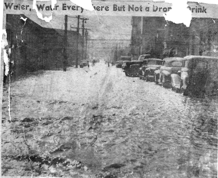
INUNDAED BY WATER FROM A BROKEN MAIN was this portion of Thirty-second St., looking toward Liberty Ave. Water seeped up through the ground and then covered the street several inches deep.
