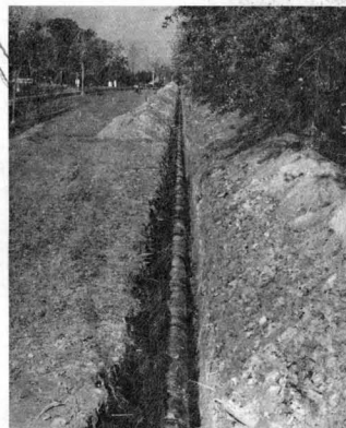
Long Straight Run of 16" Super-Lowland Pipe
