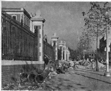
12" Pipe Being Installed Under Sidewalk
