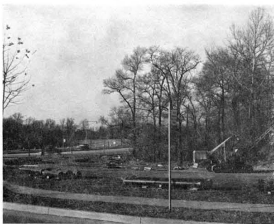
12" Pipe Strung Out Along Line of Installation
