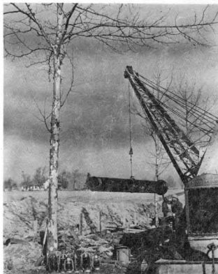
Lowering Length of 16" Pipe Into Trench
