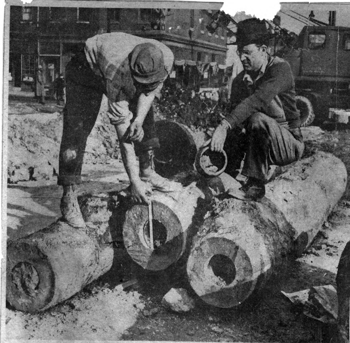
UNEARTHING TREE-TRUNK WATER MAINS ON VINE STREET
