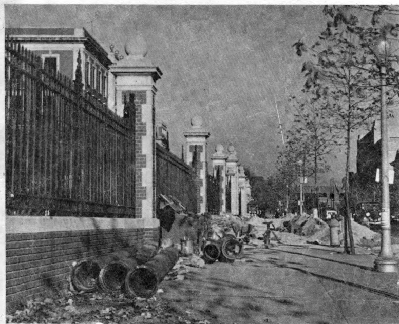
12" Pipe Being Installed Under Sidewalk
