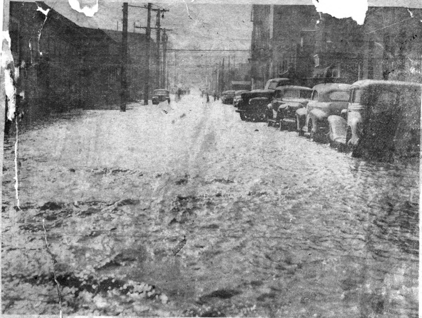
INUNDATED BY WATER FROM A BROKEN MAIN was this portion of Thirty-second St., looking toward Liberty Ave. Water seeped up through the ground and then covered the street several inches deep.
