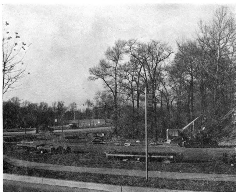
12" Pipe Strung Out Along Line of Installation
