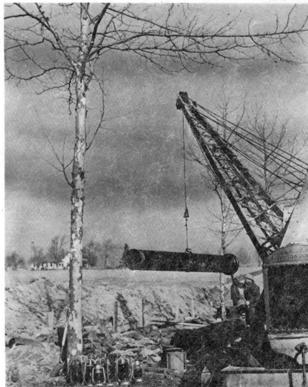
Lowering Length of 16" Pipe Into Trench
