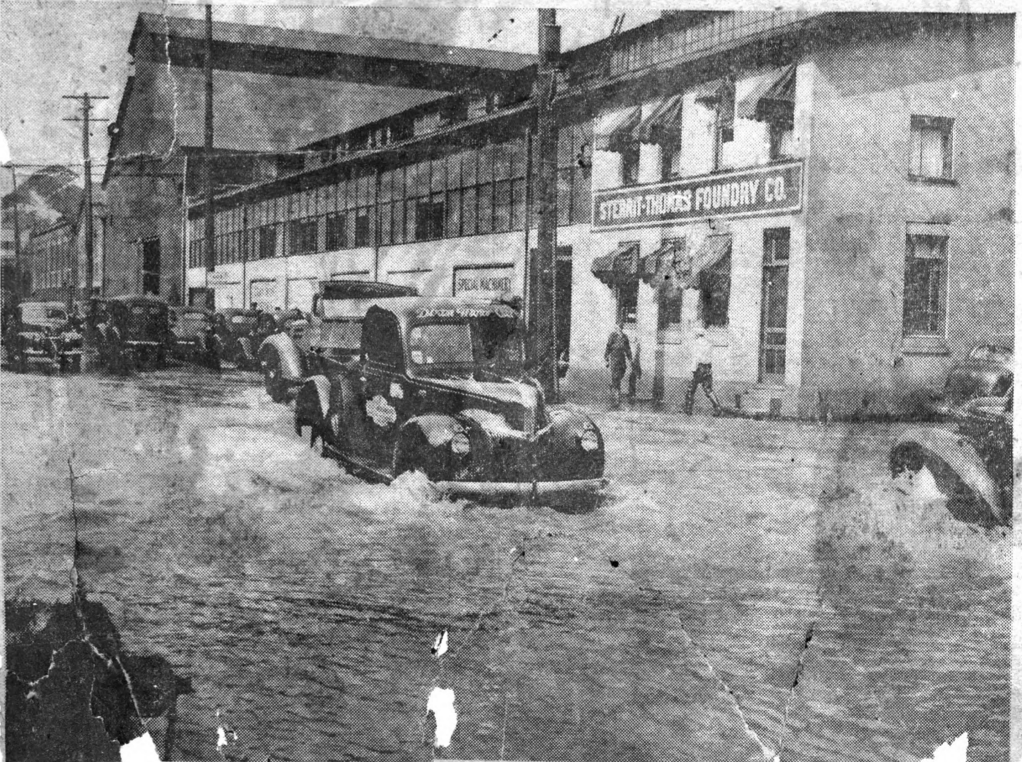
TRAFFIC MOVED SLOWLY THROUGH THE FLOOD zone at Thirty-second St., where the road was blocked off to prevent possible damage. The water gurgled up out of the ground in numerous spots and then roared down lifted curbstones six inches into the air in
