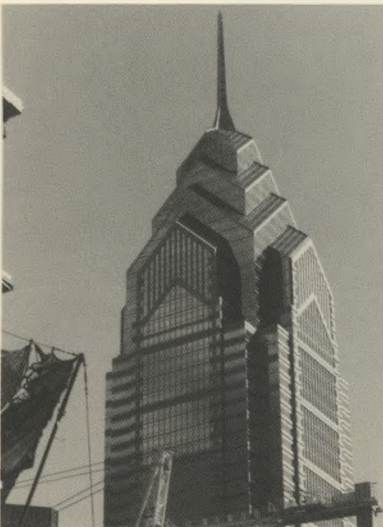
LIBERTY PLACE The construction of One Liberty Place affirms that Philadelphia is a good place to do business. Economically, it is a strong city; its big-city cultural amenities are powerful incentives which draw business and tourism.
