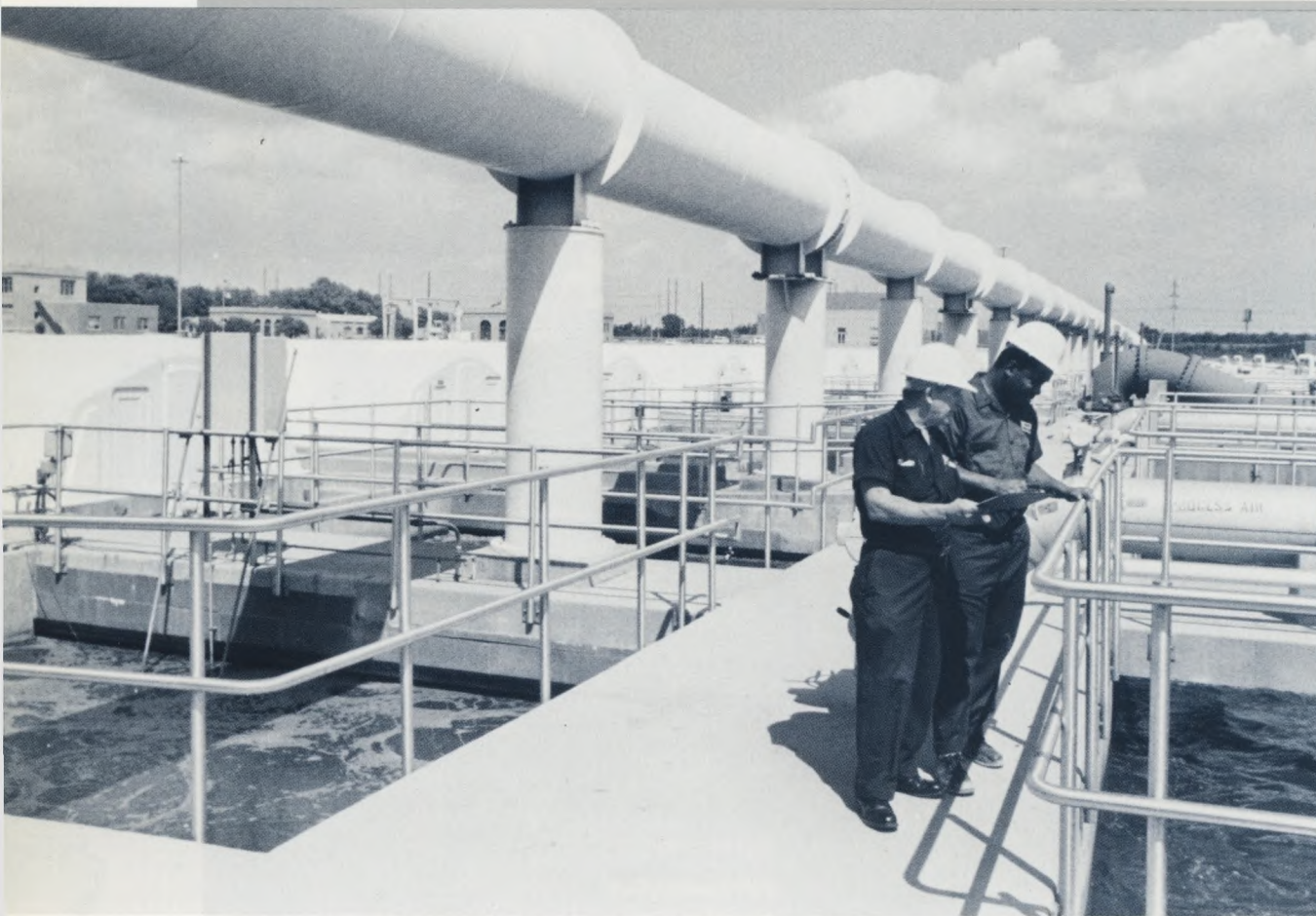
Edward Weklar and Allen Smith, Treatment Plant Operators, inspect the final sedimentation tanks at the Northeast Water Pollution Control Plant.
