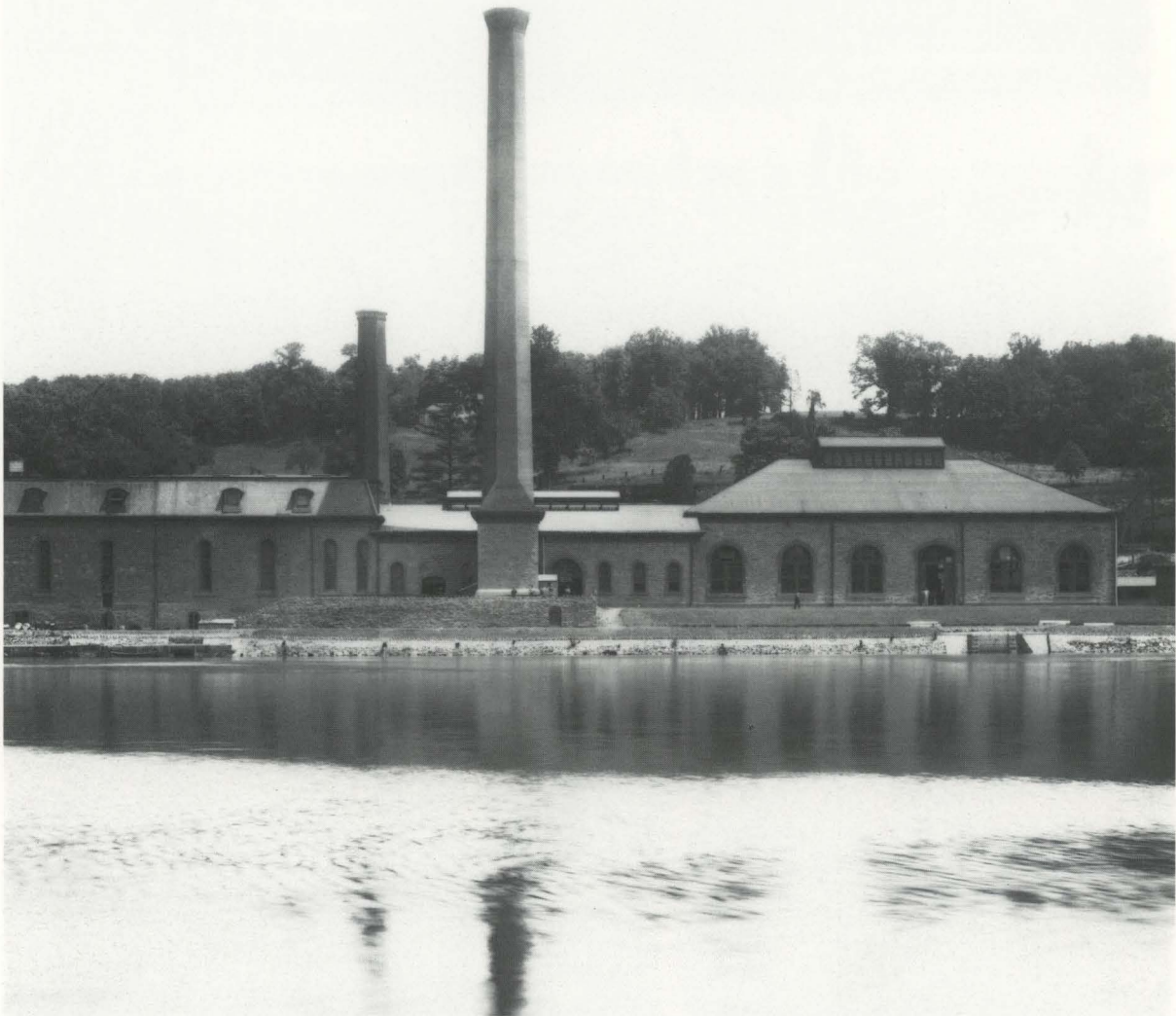
The Roxborough Pumping Station, built in 1866, originally supplied the Roxborough, Manayunk and Germantown sections of the City with raw river water. It was later refurbished in 1903, as pictured here, and renamed the Shawmont Pumping Station.
