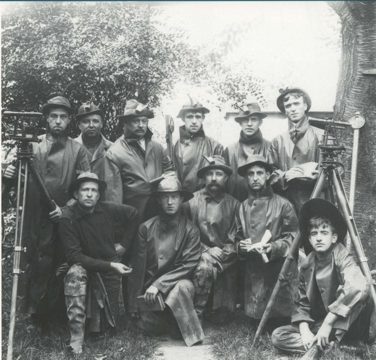
A Survey crew was pictured in 1903, during their assignment to survey the construction of the Torresdale Conduit, which was built through rock 100 feet below the surface. The conduit was approximately three miles long and 12 feet in outside diameter and connected the Torresdale Filtration Beds to the Lardner's Point Pumping Station.
