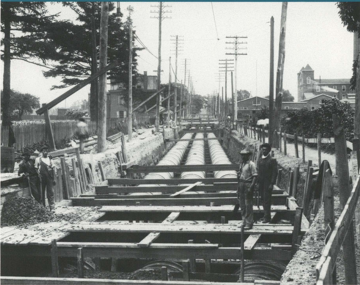
New distribution mains were laid along State Road in 1904 to supply the Northeast section of the City with filtered water from the Lardner's Point Pumping Station.
