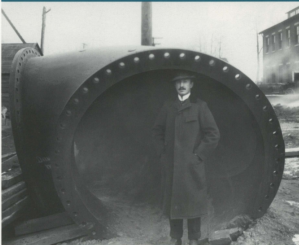
The construction of the Lardner's Point Pumping Station in 1903 included the installation of six foot diameter cast iron pipe sections used to connect valve chambers for the distribution of filtered water.
