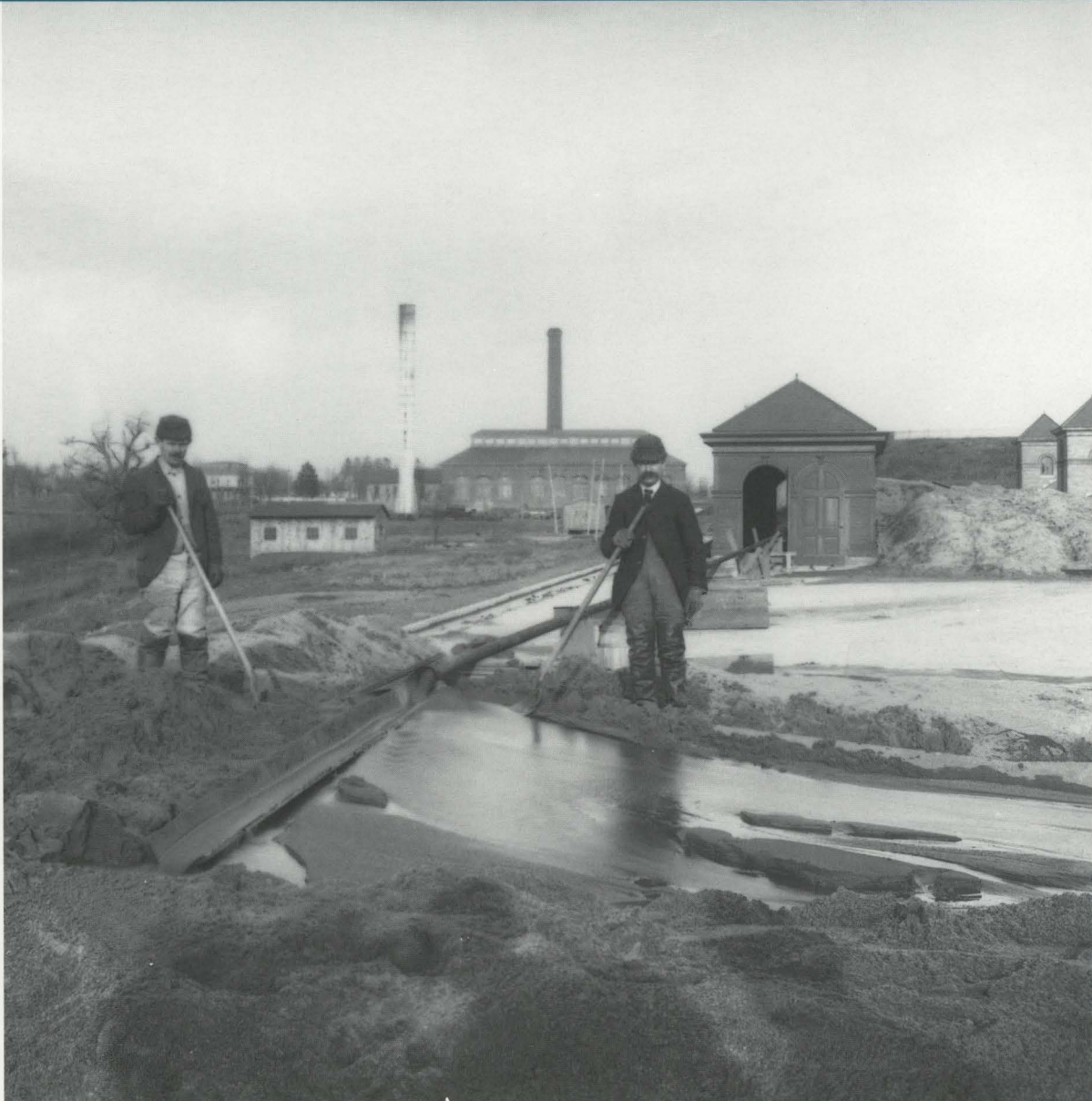
Preparing for the start-up of the Upper Roxborough Filter Beds in 1903 included the storage of large quantities of sand in the court area of the underground filter beds.
