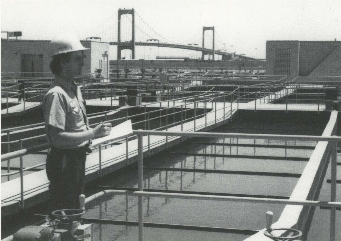
Operator checks one of the twelve final sedimentation tanks at the new Southeast Water Pollution Control Plant, which hold a total of 14.4 million gallons.
