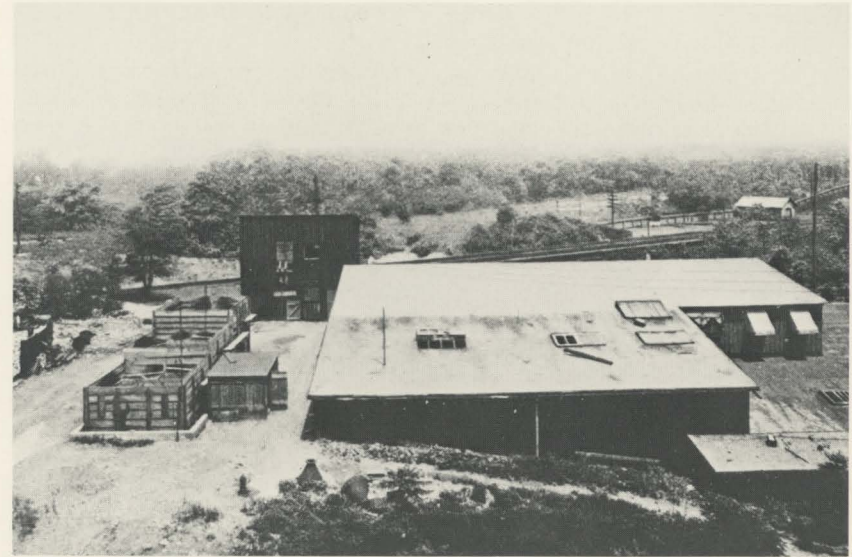
SPRING GARDEN STATION: At this humble facility, Philadelphia made its first experiments with sewage treatment from April 1, 1909 to April 30, 1910. A half-dozen different methods were tried.
