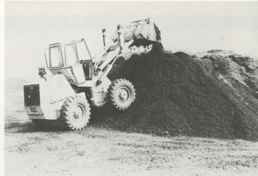
COMPOSTING: A front end loader (above) mixes wood chips with the dewatered sludge cake prior to the delivery to large compost piles. A forced aeration compost method is used. The composted sludge is screened (below) to remove the bulking agent (wood chips) which is reused.
