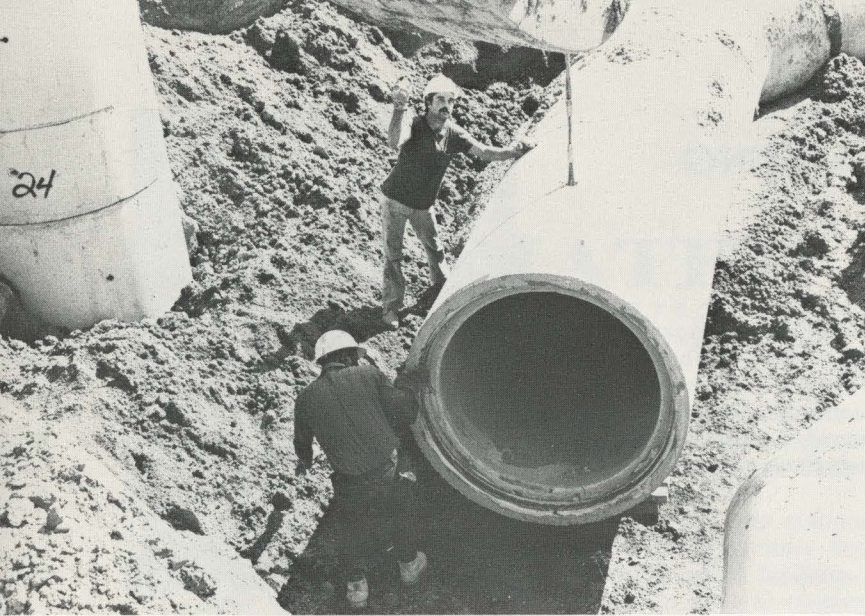
PRECAST CONCRETE PIPE: This type of pipe has replaced the use of old brick sewers to drain storm water from newly developed areas in Philadelphia.
