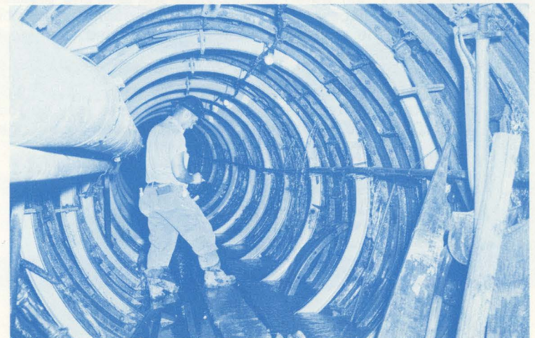
Of 150 miles of sewer interceptors, the city has added 80 miles in recent years. The big interceptors pick up mixed flows from branch sewers and carry them to plants for treatment. Map shows expansion; photo below, an interceptor on the west bank of the Schuylkill River.
