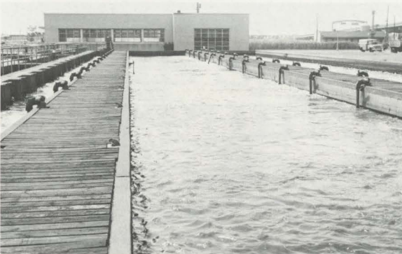
FLOCCULATION: Blown from diffuser tubes, air is bubbled through the flow in the 250-ft. long tanks above at the Southeast Plant. Such air injection helps to float grease and coagulate particles in both "primary" plants.
