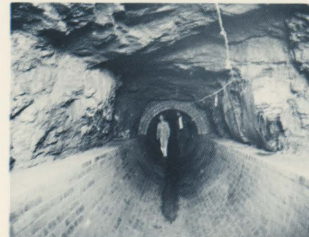
BRICK GIANT: Many large brick sewers were built by Philadelphia in the late 19th century and the early 20th. This large sewer, constructed in 1917, was one of the last big brick lines created.
