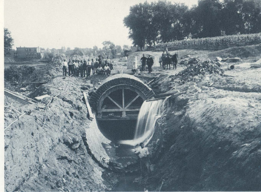
LEGACY OF THE PAST: Typical of old brick sewers built at the turn of the century was this 1909 sewer in Fairhill Street, intended to enclose Rock Run. Today the city is spending $8-$10 million a year to replace 600 miles of these brick veterans. One replacement (in Belfield Avenue) is shown below.
