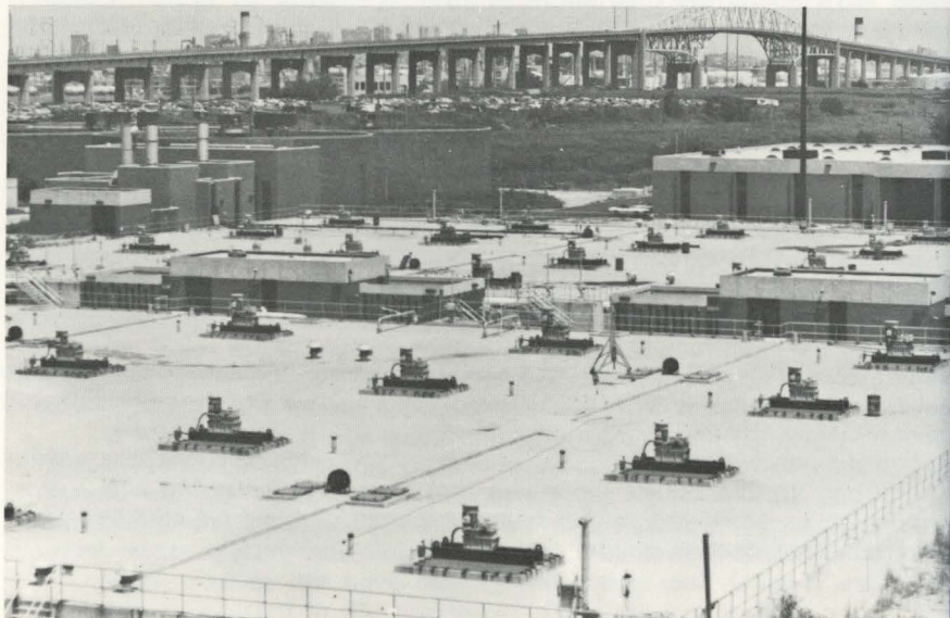
SOUTHWEST PLANT: Expansion to a 210 million gallon per day, oxygen activated sludge plant is virtually complete. Foreground above shows half of the twenty rectangular final sedimentation tanks. Seen below are the aeration tanks which are covered to confine the oxygen rich atmosphere above the water surface.
