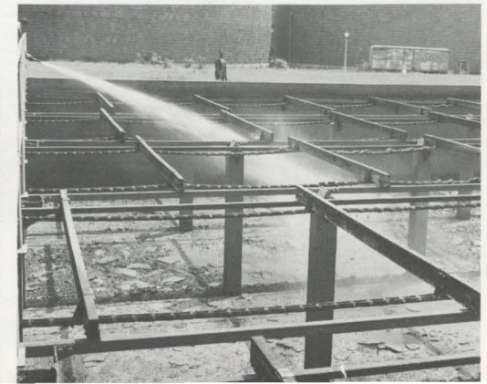
GRIT REMOVAL: After screening, the wastewater flows through the 50-ft. channels (top photo), and there the grit settles out and is removed by chain operated "collectors" to the screw conveyor (lower photo).
