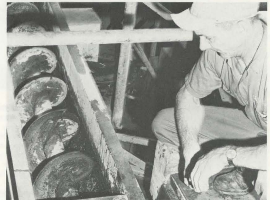
GRIT REMOVAL: After screening, the wastewater flows through the 50-ft. channels (top photo), and there the grit settles out and is removed by chain operated "collectors" to the screw conveyor (lower photo).
