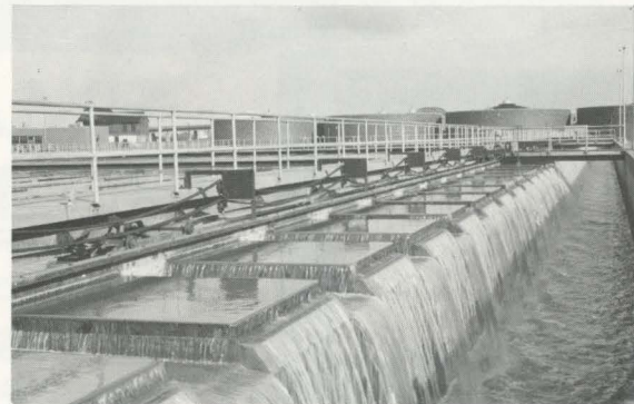
EFFLUENT: After removal of part of the solids, the effluent, or liquid, flows to the secondary process.
