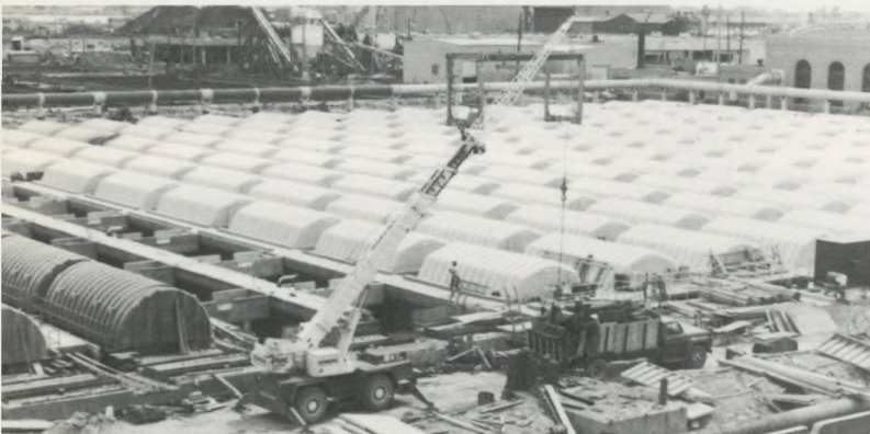
Rows of fiberglass shells cover the 280 rotating biological contactors as they are installed (right) in the aeration tanks at the Northeast Water Pollution Control Plant.
