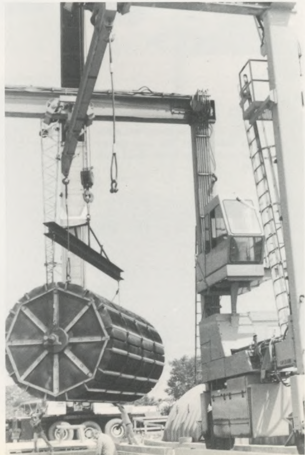
Rows of fiberglass shells cover the 280 rotating biological contactors as they are installed (right) in the aeration tanks at the Northeast Water Pollution Control Plant.
