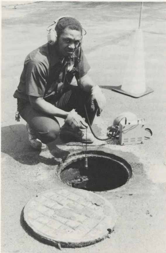
The Detect-A-Leak Unit lets Milton Fletcher, Water Distribution Repairman, listen to water main valves, fire hydrants and service lines to find leak noise. Plugging the unit into the van-mounted computer allows the leak to be pinpointed with accuracy.
