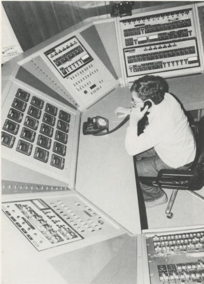
Water System Load Control Dispatcher Alexander Karczewski keeps our energy costs down by pumping more water at night.
