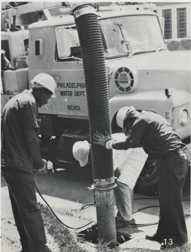
The city's 75,000 inlets are a constant challenge to clean-up crews. Many can be cleaned by crane; others require a special vacuum truck (below).
