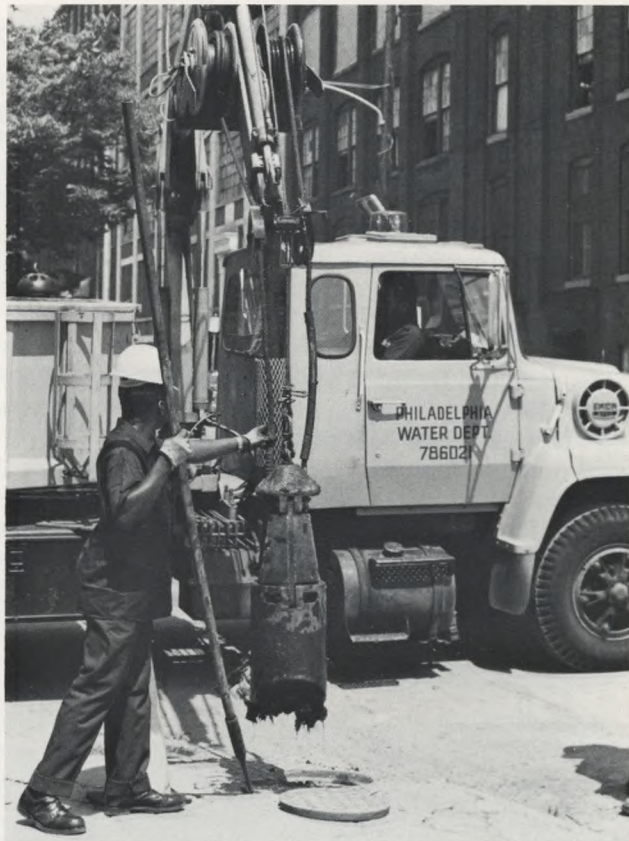
The city's 75,000 inlets are a constant challenge to clean-up crews. Many can be cleaned by crane; others require a special vacuum truck (below).
