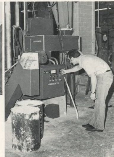
Lime Feed: Old problems caused by lime dust and the settling of lime in conduits and basins were eliminated at the Torresdale Water Plant, when new lime feeders, slakers, and dust collectors were installed.
