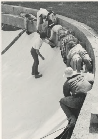
Reservoir Cover: Workmen place a gigantic floating cover of synthetic rubber on the north basin of the Oak Lane Reservoir. The Water Department plans to cover all its open reservoirs to protect purified water from algae and contamination.
