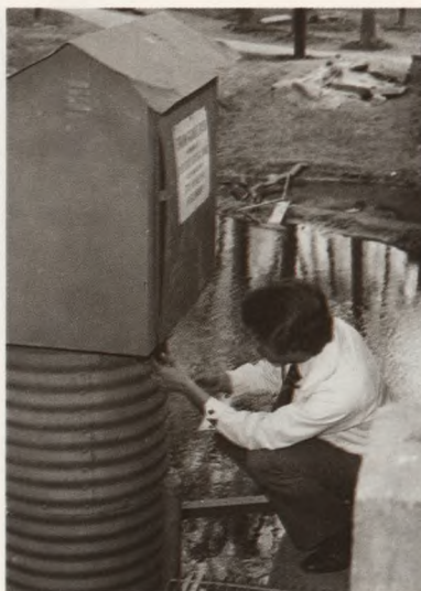
Stream Gauge: Flow rates and water volumes were measured in creeks by a network of stream gauges. The Water Department maintains such gauges to study the pollutional effects of urban runoff.
