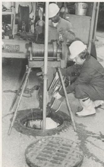
For Efficient Sewers: Crews inspected 207 miles of sewers by walking, crawling, or hauling a television camera. They also cleaned sewers and installed a new type of locking nut on inlet covers.
