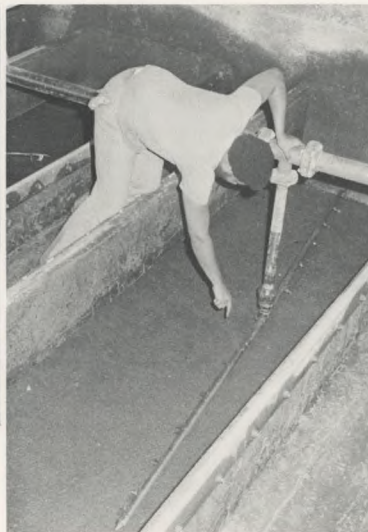
High Rate Study: Equipment for adding coagulant chemicals and recording flow rates, etc., is inspected at the site of a Neptune microfloc filter. If high rate filters prove successful, all filter beds at Queen Lane will be converted to high rate filtration.
