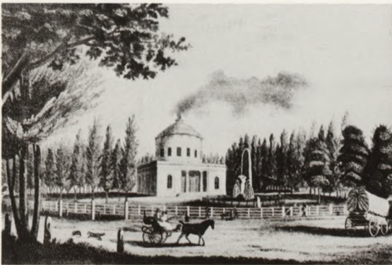
The first use in America of steam pumps for large scale water supply began in Philadelphia in 1801. A Schuylkill River station (above) pumped water to a station at Centre Square (below). This early system was the work of Benjamin Henry Latrobe.
