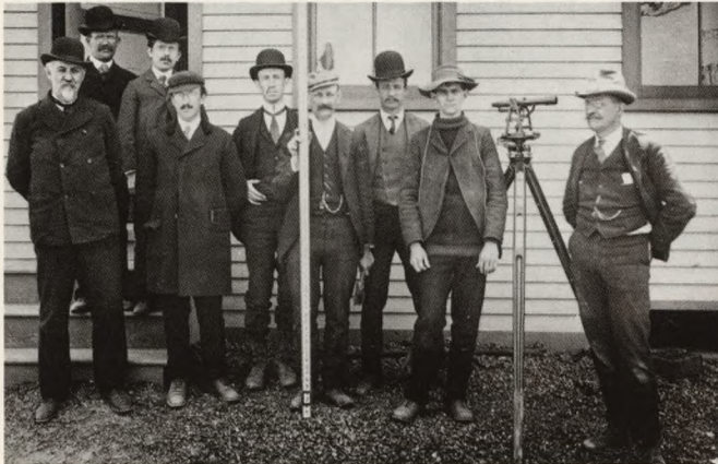
In Days of Yore: Surveyors used a sighting instrument and calibrated rod to survey lines for water mains, sewers, and other city projects. Distinguished group posed for this photograph in 1903.
