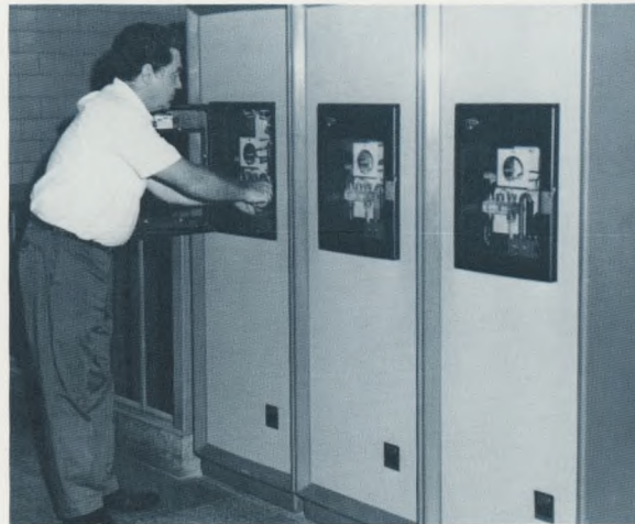
For Better Water: An operator checks the control panel (right) of a new ammoniation system at the Torresdale Plant. Ammonia will be used to remove chlorinous tastes and odors from finished water. Photo at left shows ammonia applicators.
