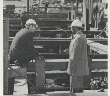
New Sewers: Twenty-three miles of new sewers were built during the biennium in all parts of the city.
