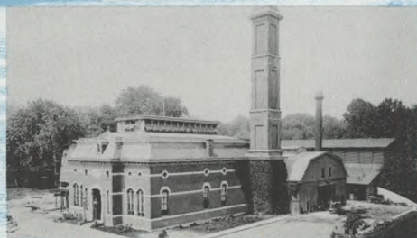
Steam pumping stations grew bigger. Belmont (1872).
