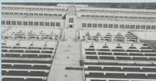
Covered filter beds extended over 60 acres at original 1905 Torresdale Plant.
