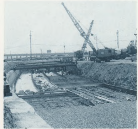
Sewers for Eastwick: Many huge storm water lines were built to serve new homes in the redeveloped Eastwick area. Photos show construction of a four-cell conduit of reinforced concrete in Bartram Ave. Each cell measures 7 ft. x 11½ ft. in size.
