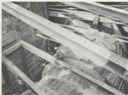
Mill Creek Sewer: A perilous reconstruction job, the new sewer was built at depths of 40 feet while maintaining a heavy flow.
