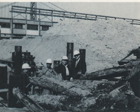
Sewer Replacement: Many miles of old brick sewers were replaced with new concrete lines. Two of the most unusual were century-old storm water sewers with wooden bottoms, emptying into the Delaware River at Market St.
