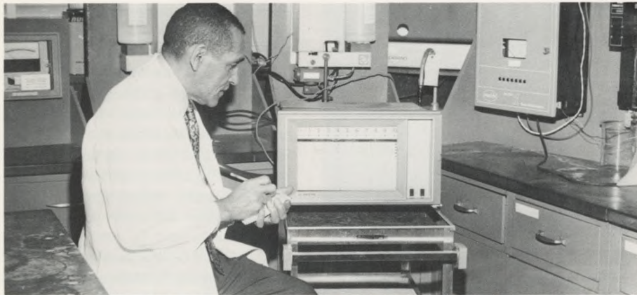
Towards Automation: Plant laboratories experimented with new types of automated testing devices, in order to reduce time-consuming wet chemical tests. The new devices were proving fast and efficient.
