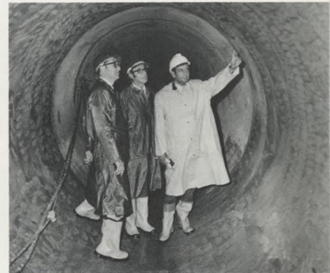
Water Abundance: The new tunnel will carry up to 150 million gallons of river water daily, assuring plenty of water to meet growing demand.
