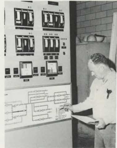
For Better Water: An operator checks the control panel (right) of a new ammoniation system at the Torresdale Plant. Ammonia will be used to remove chlorinous tastes and odors from finished water. Photo at left shows ammonia applicators.
