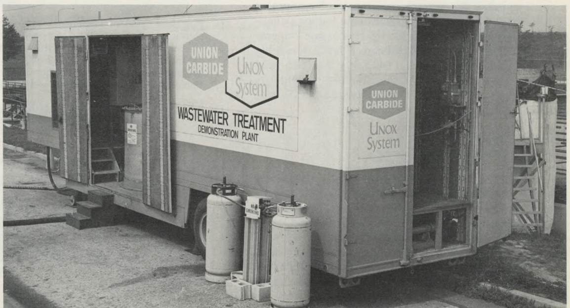
Treatment Experiment: Looking for new ways to improve plant efficiency, the Water Department injected pure oxygen (instead of air) into an aeration tank at the Northeast Plant. The experiment, conducted from the trailer, indicated a marked improvement in the destruction of wastes by aerobic bacteria.
