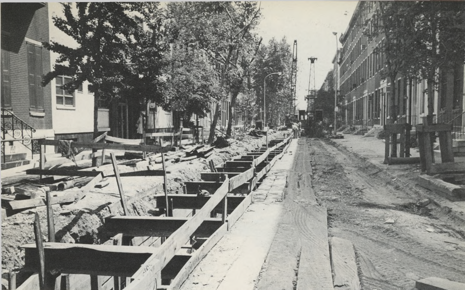
Old Sewers: Replacement of a 140-year old brick sewer in Pine Street was one of the largest sewer jobs. The line was being replaced for several blocks with a new reinforced concrete conduit, as part of a continuing program to remove deteriorating sewers. Pine Street job, above and below.
