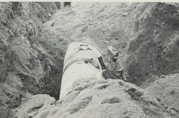
Broad Street Link: Remarkable for its bends and curves, a new steel water main was laid around the east side of City Hall to serve as a link in the huge Broad Street supply line. Workmen make a cross-tie at right and seal the main below.
