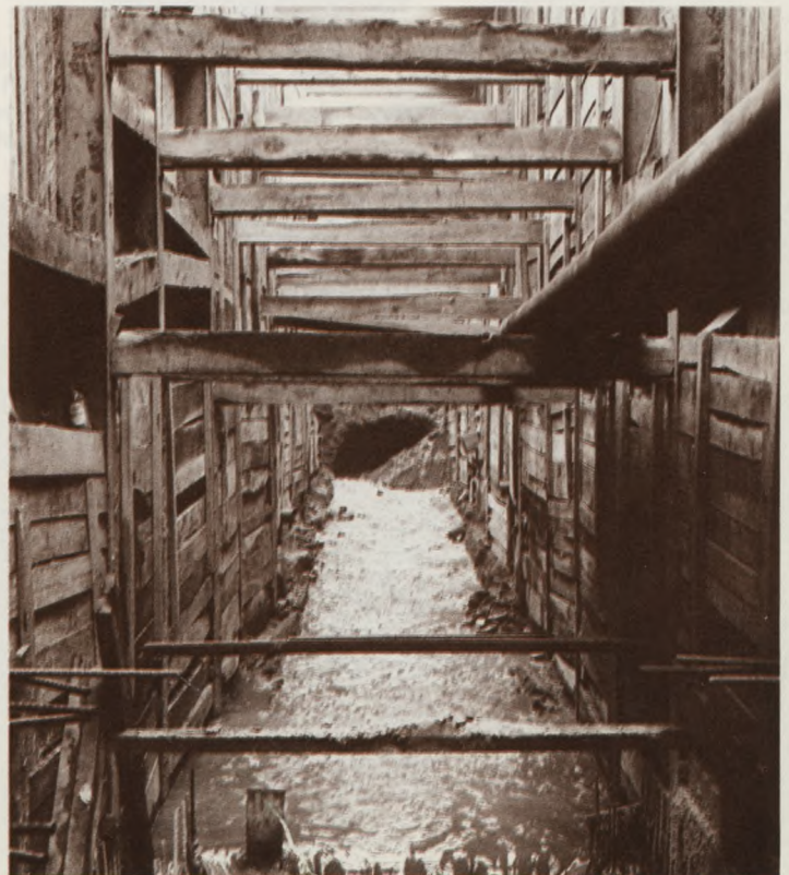
Old Sewers: Replacement of a 140-year old brick sewer in Pine Street was one of the largest sewer jobs. The line was being replaced for several blocks with a new reinforced concrete conduit, as part of a continuing program to remove deteriorating sewers. Pine Street job, above and below.
