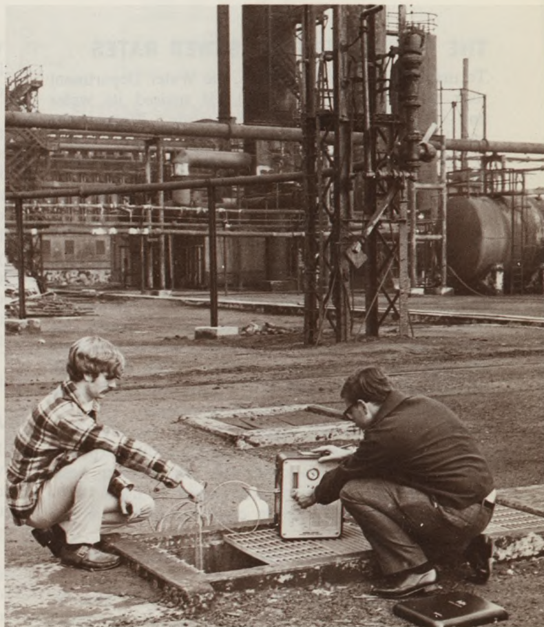
New Surcharge: As part of an enforcement program for a new surcharge on industrial wastes, sanitary engineers monitored the wastes of many industries in 1970-71. Above, department engineers take "readings" on waste discharges into city sewers by two industries.
