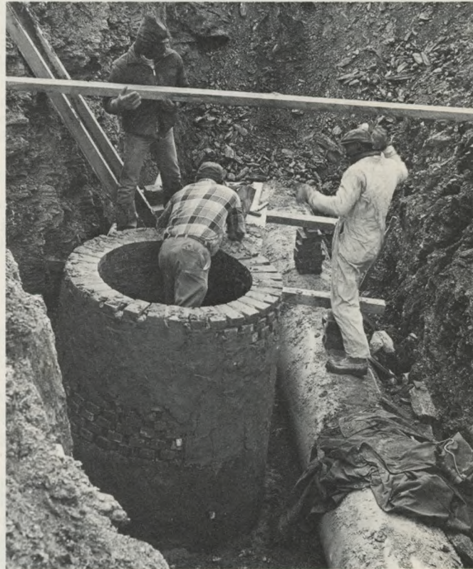
In the Northeast: To meet the needs of new homes, a sewer is laid (left), while workmen build a related manhole (below). Nine miles of sewers were built in all parts of the city during the biennium to service newly developed or redeveloped neighborhoods.
