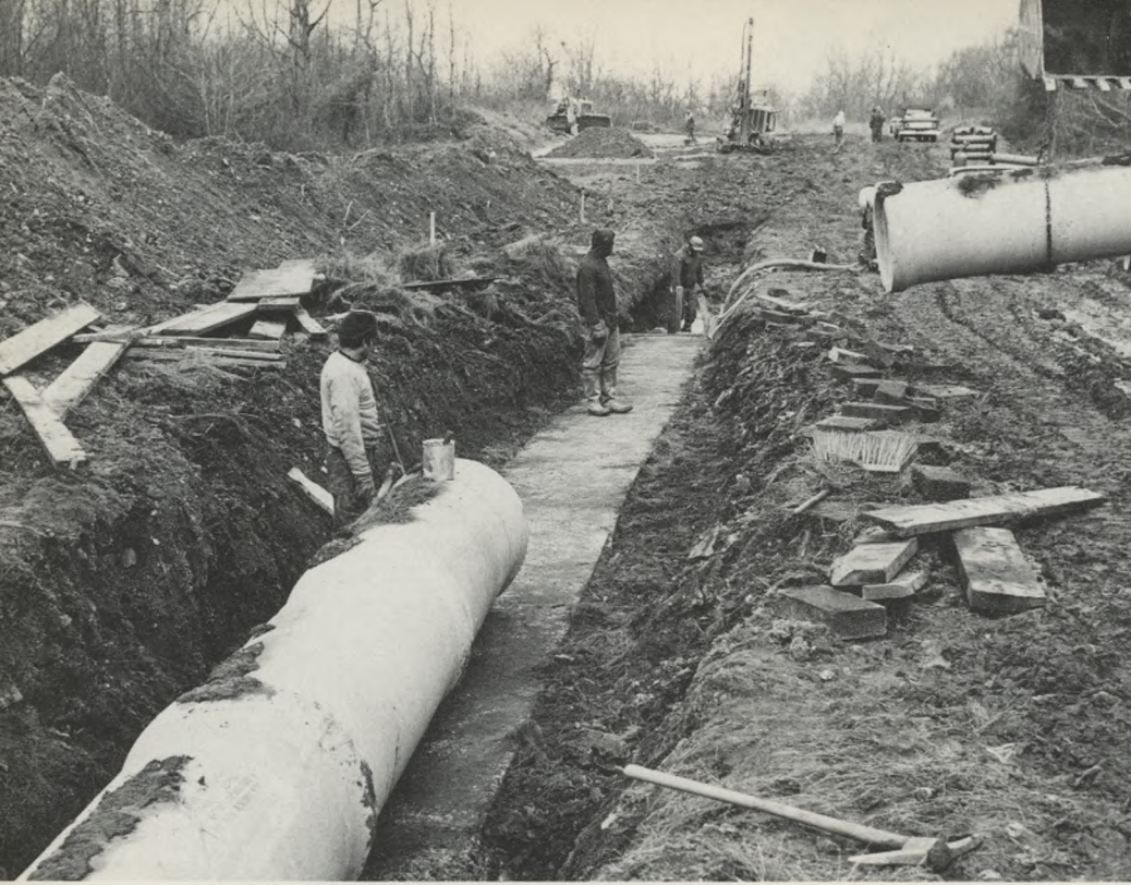
In the Northeast: To meet the needs of new homes, a sewer is laid (left), while workmen build a related manhole (below). Nine miles of sewers were built in all parts of the city during the biennium to service newly developed or redeveloped neighborhoods.
