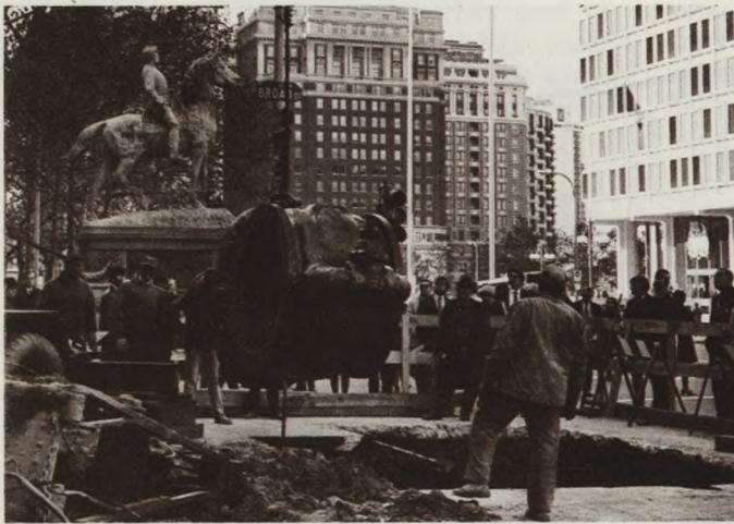
... Replace Hundreds of Miles of Old Deteriorating Water Mains and Sewers
