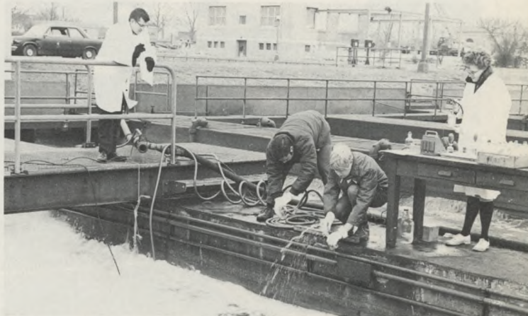
For More Efficient Treatment: Two new mechanical aerators went into service (below) at the Northeast Plant, supplementing the air supplied by blowers to the aeration tanks. Chemists (above) check effect of additional aeration on the wastewater being treated. Air is needed by aerobic bacteria to break down wastes in the tanks.
