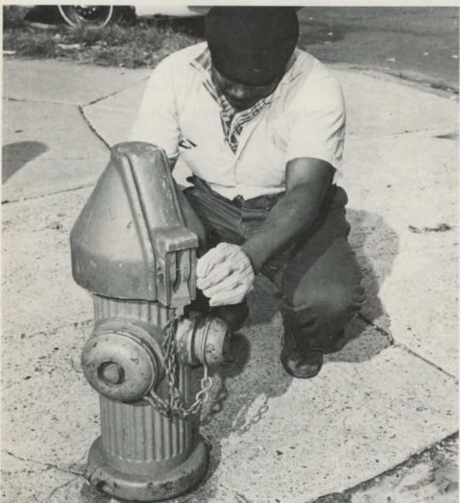
Locking Bonnet: In addition to the locking nut, the Water Department experimented with a special security bonnet (above). Removable only with a special tool (below right), the bonnet may prevent illegal hydrant openings.
