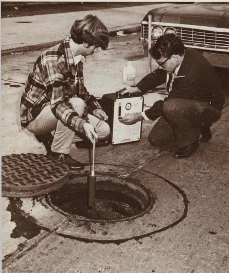
New Surcharge: As part of an enforcement program for a new surcharge on industrial wastes, sanitary engineers monitored the wastes of many industries in 1970-71. Above, department engineers take "readings" on waste discharges into city sewers by two industries.
