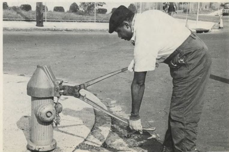
Locking Bonnet: In addition to the locking nut, the Water Department experimented with a special security bonnet (above). Removable only with a special tool (below right), the bonnet may prevent illegal hydrant openings.
