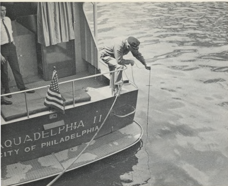
On-board Analyses: Equipped with an on-board laboratory (photo below), the department's new cabin cruiser allows sanitary engineers to study river water samples while afloat. Samples are drawn through the bottom of the boat, flowing out through laboratory faucets, or they are collected by brass container and bottle dropped overboard, as shown above.
