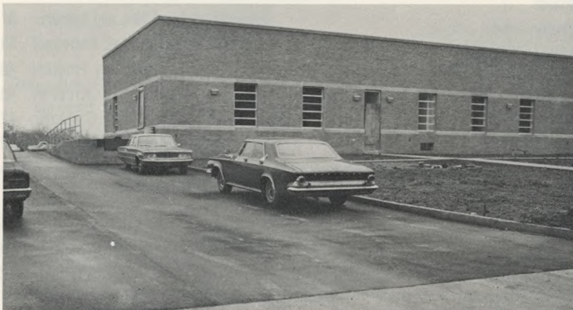
At the Queen Lane Plant a new building, with automatic equipment, augured further improvements in the city's water.
