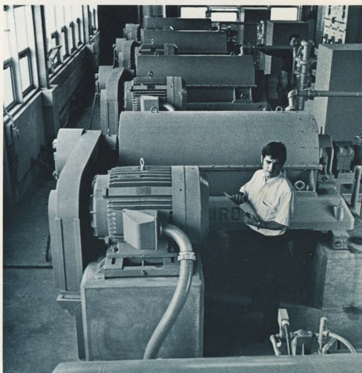
For Dewatering Sludge: An $804,000 station was built at the Southwest Plant to remove some of the water from digested sludge. Five steel centrifuges (below) will whirl the sludge. Because digested sludge is barged to sea, a less watery sludge will save the city money.
