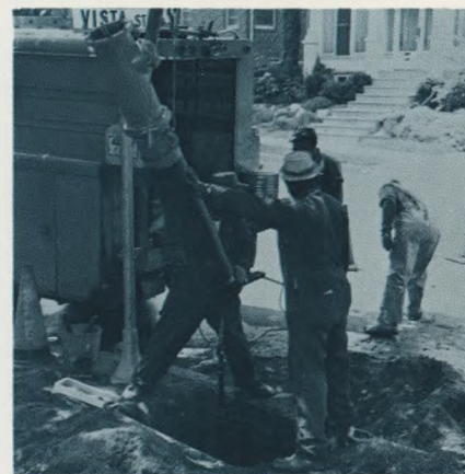
New Fire Hydrant: A hydrant is lowered into place in a residential neighborhood. It is one of 25,000 such hydrants that protect the city.
