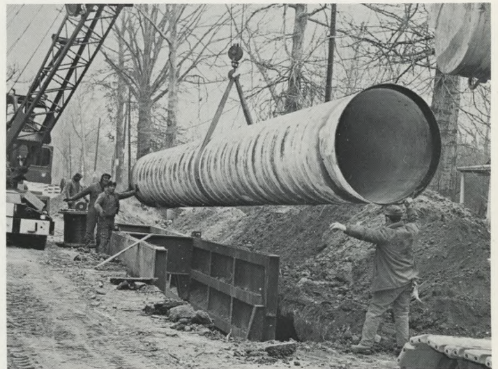
With Federal Aid: Four feet in diameter, the steel main moved steadily northward on State Road. The Federal Government agreed to pay 45% of the $1 million price tag.
