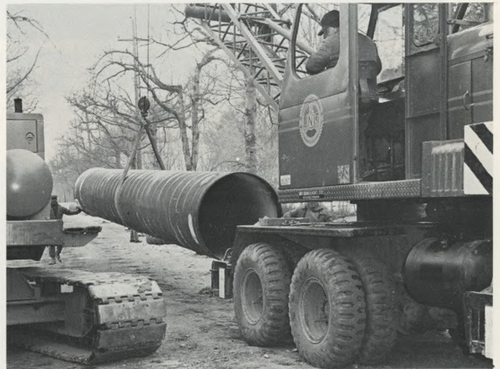
With Federal Aid: Four feet in diameter, the steel main moved steadily northward on State Road. The Federal Government agreed to pay 45% of the $1 million price tag.
