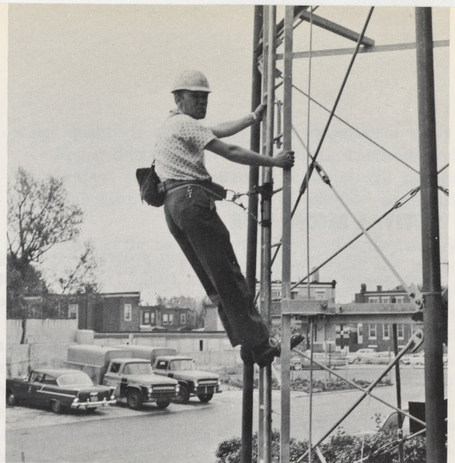
For Safer Climbing: The safety program was tightened as installation of a new safety device began at microwave towers and water tanks. Attaching himself to a sliding piece which rode on a pipe-like rail with fall-breaking notches, the climber could be much safer.
