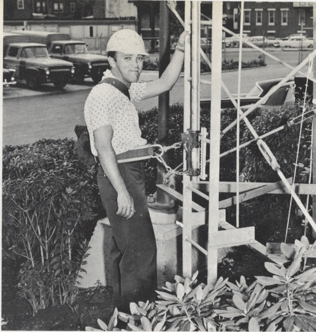
For Safer Climbing: The safety program was tightened as installation of a new safety device began at microwave towers and water tanks. Attaching himself to a sliding piece which rode on a pipe-like rail with fall-breaking notches, the climber could be much safer.
