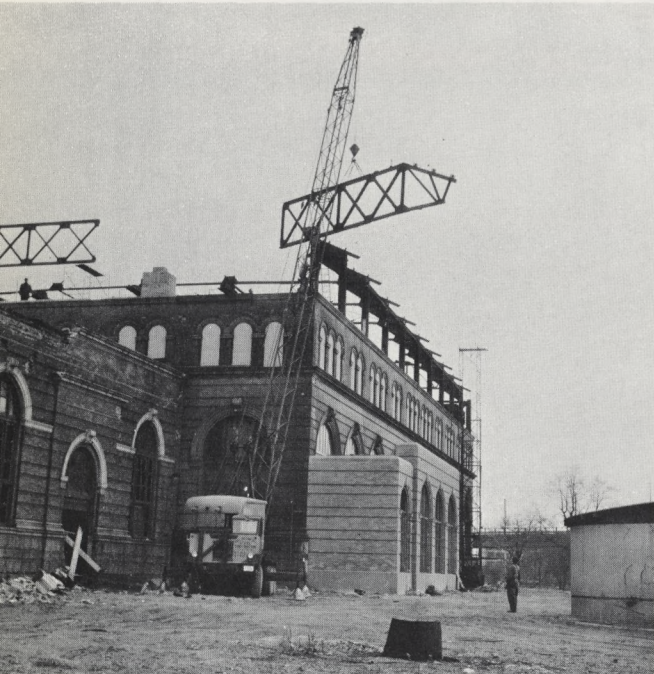
Lardner's Point: The City's largest filtered water pumping station was undergoing its final face lifting as part of a $3.4 million modernization dating back many years. Cranes removed the old roof of the station's single remaining building, and extensive renovations were made.
