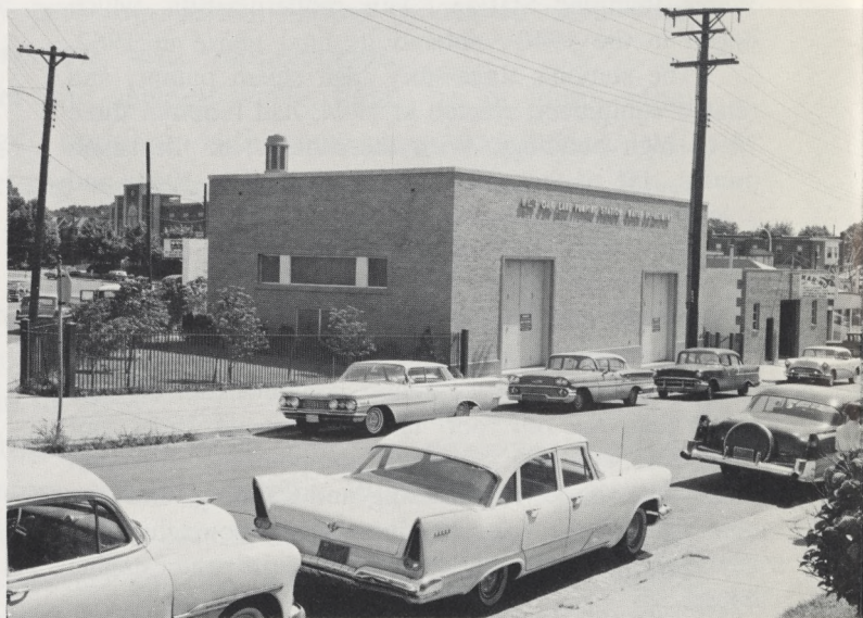
A New Pumping Station: The new West Oak Lane Station, which opened in April, is operated by microwave from the Water Department's microwave control center. With pumping capacity of 27 million gallons daily, it pumps Torresdale Plant water into the Northwest.
