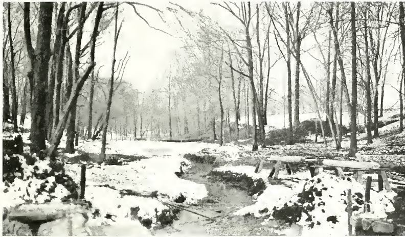
ONE OF THE FIRST OF CAMDEN COUNTY'S PARKS NOW UNDER CONSTRUCTION— THE MUNN MEADOW SECTION OF SPRING BROOK VALLEY.
