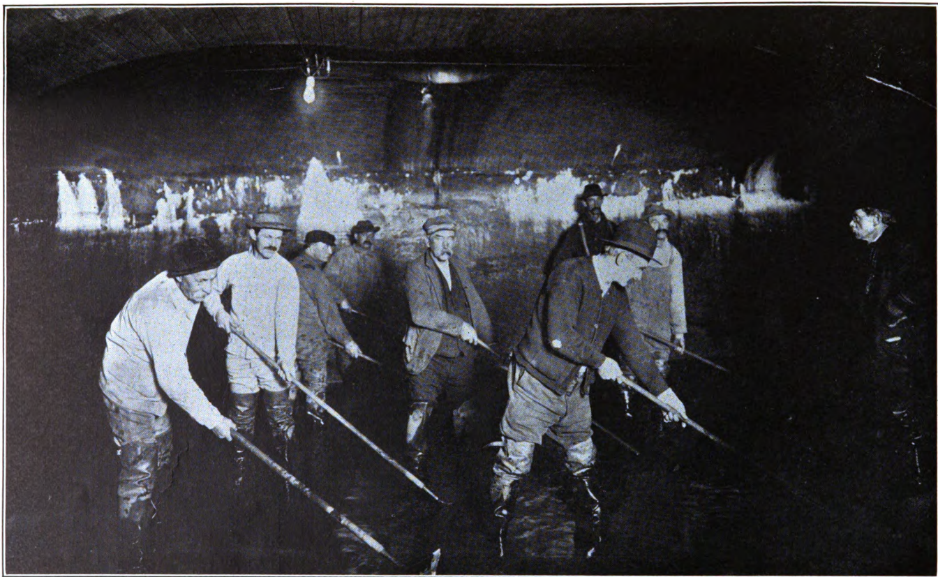
Cleaning Filters. "Brooklyn" Method.
