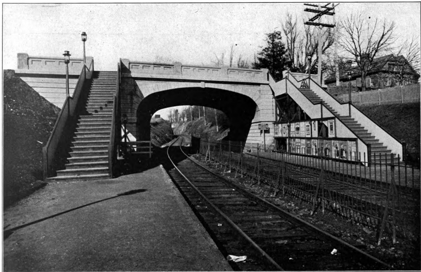
GRAVERS' LANE BRIDGE OVER CHESTNUT HILL BRANCH PHILADELPHIA & READING RAILWAY.
