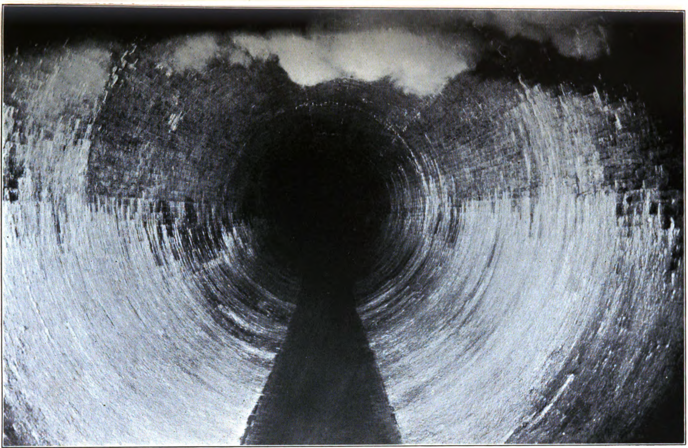
PLATE NO. 9.—LINING OF TUNNEL UNDER SHAFT NO. 8.
