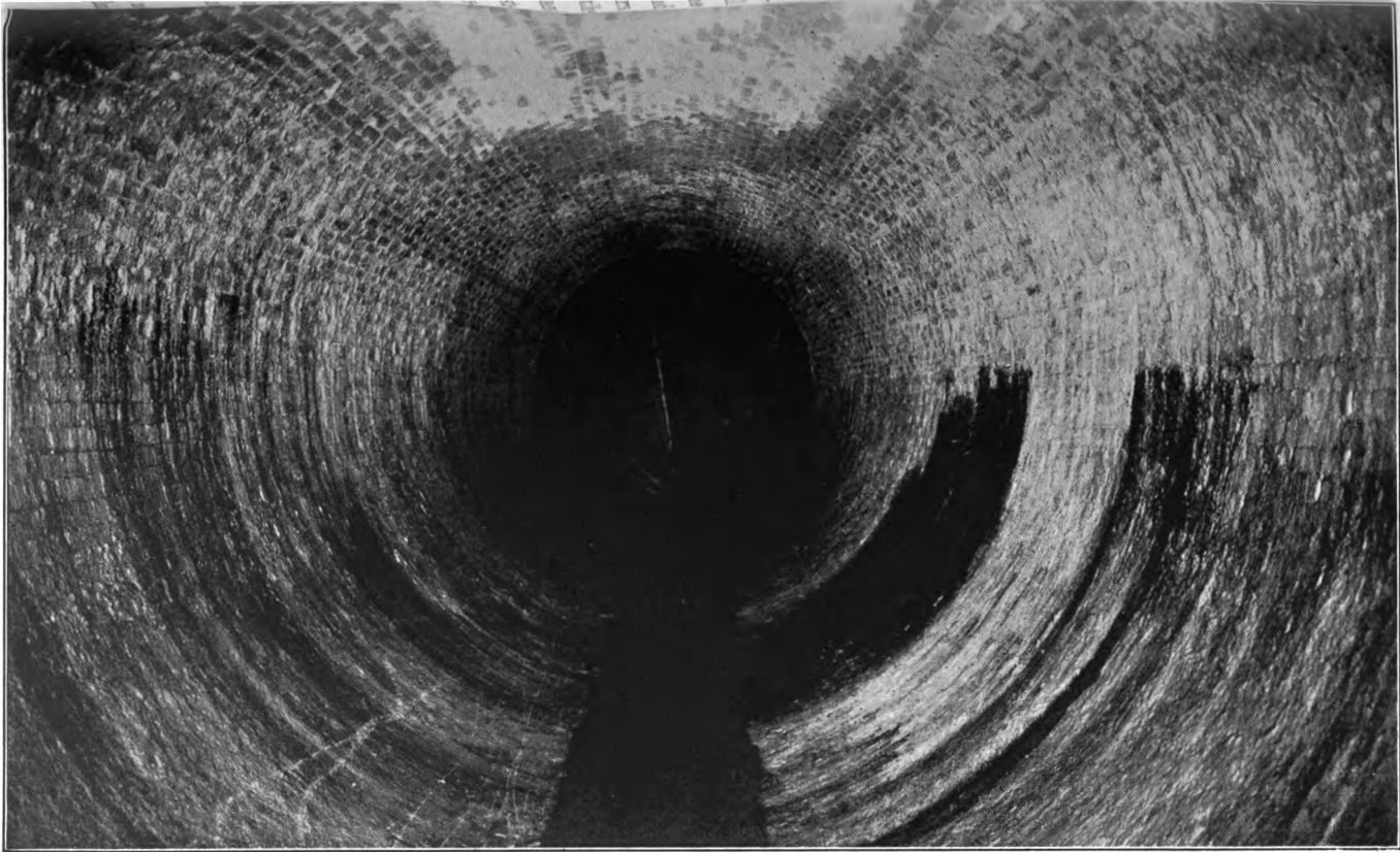
PLATE NO. 12.—LINING OF TUNNEL AT FOOT OF SHAFT NO. II.
