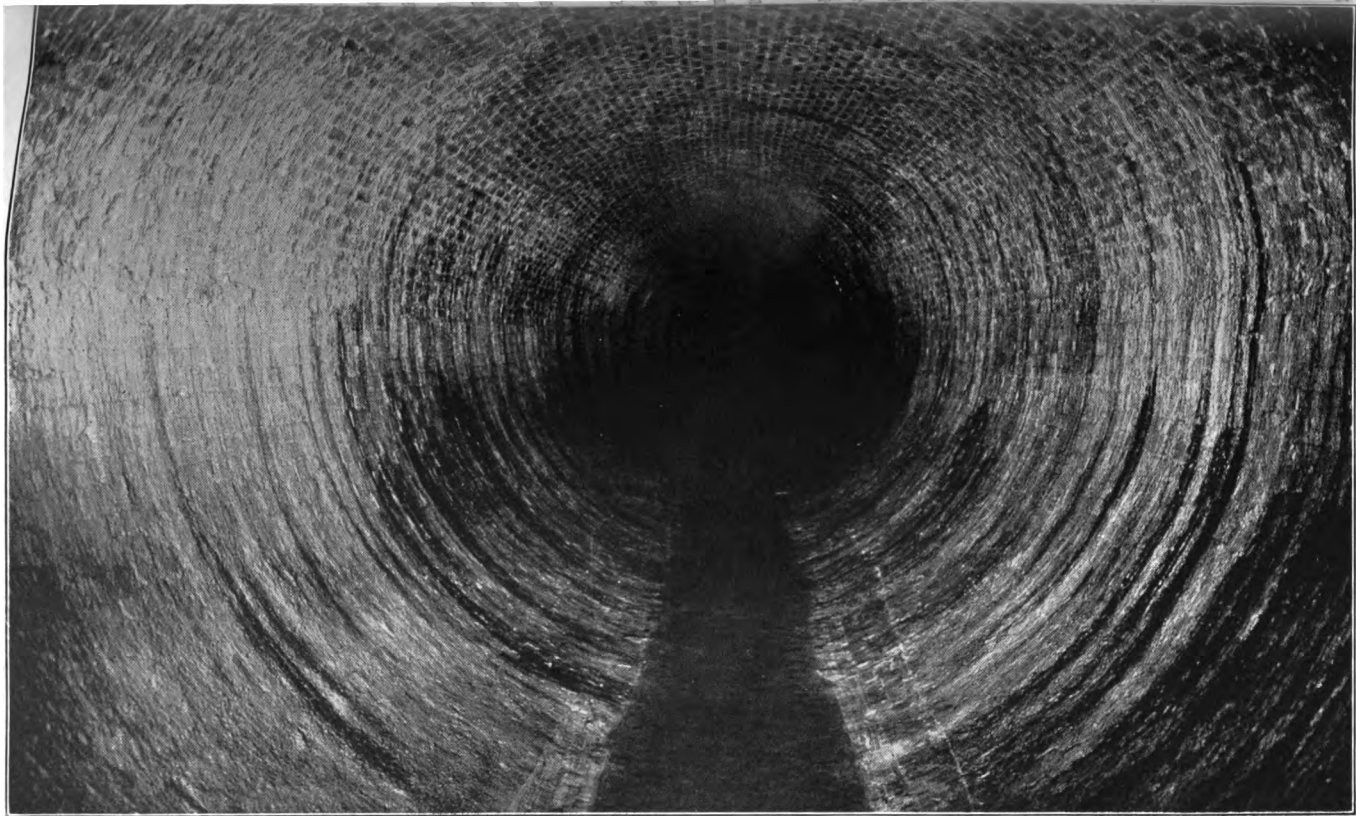
PLATE NO. II.—LINING OF TUNNEL UNDER SHAFT NO. 10.
