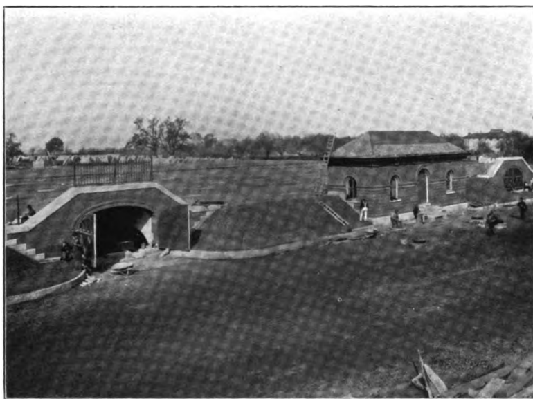
FIG. 9.—UPPER ROXBOROUGH FILTERS—FILTER ENTRANCE AND REGULATOR HOUSE.
