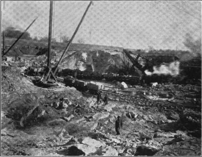
FIG. 4.—BELMONT RESERVOIR EXCAVATION—WEST BASIN.
