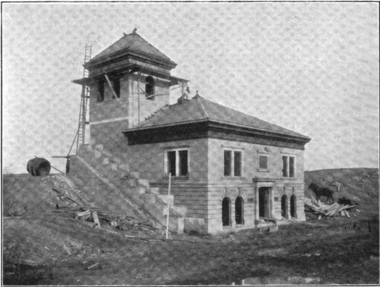
FIG. 6.—BELMONT RESERVOIR—INLET AND OUTLET GATE HOUSE.
