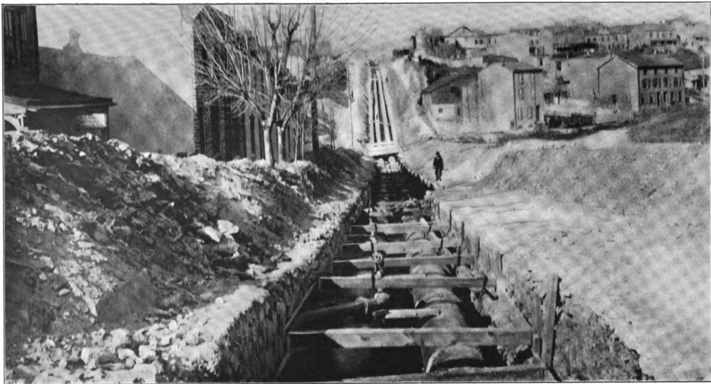
DOUBLE LINE 30" PIPE, SILVERWOOD STREET. NOVEMBER 8, 1901.
