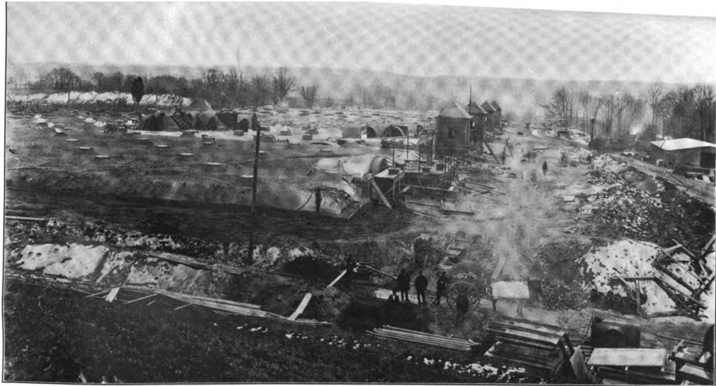
LOWER ROXBOROUGH FILTER PLANT. JANUARY 14, 1902.
