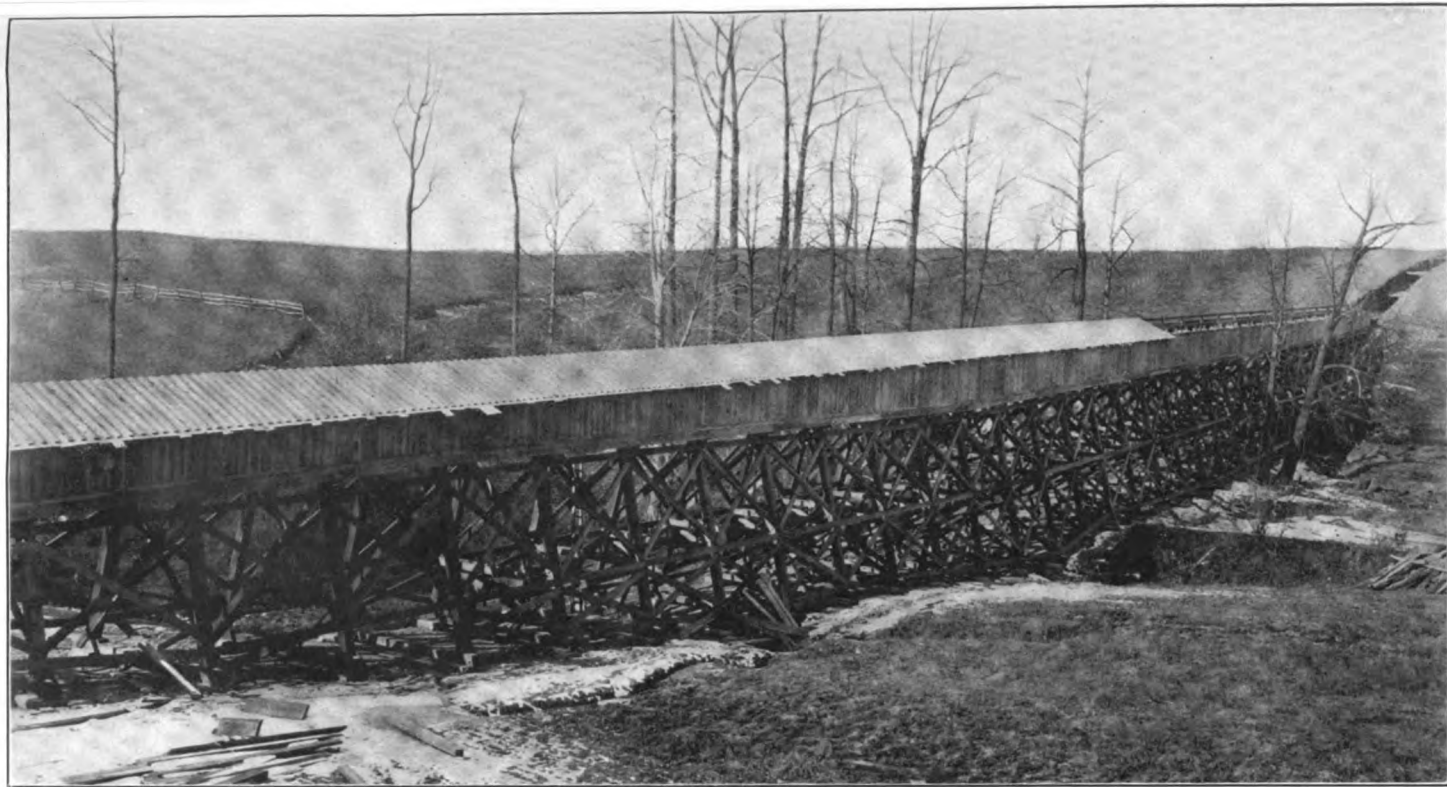
Two 30" WATER MAINS, SILVERWOOD STREET. JANUARY 18, 1902.
