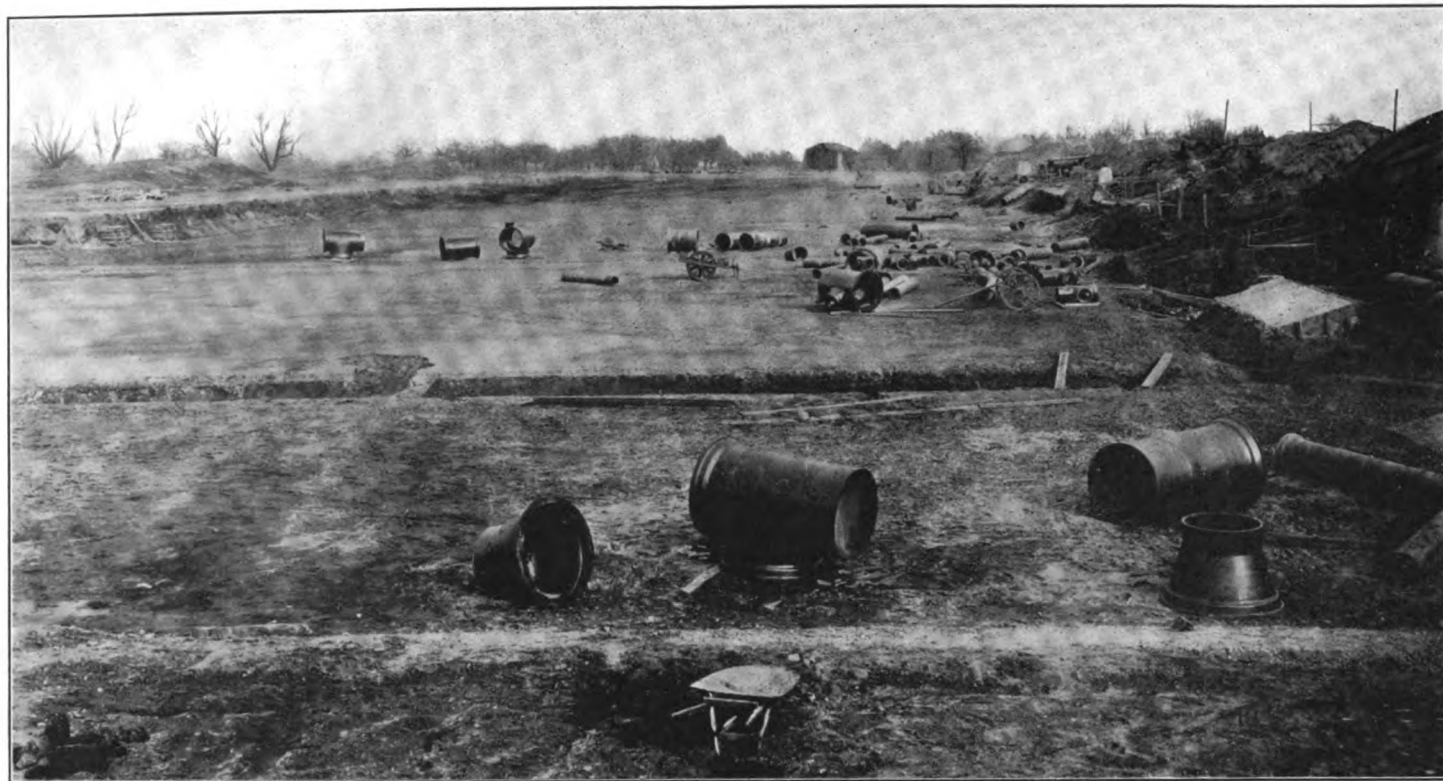
EXCAVATION FOR FILTERS, UPPER ROXBOROUGH FILTERS. JANUARY 7, 1902.
