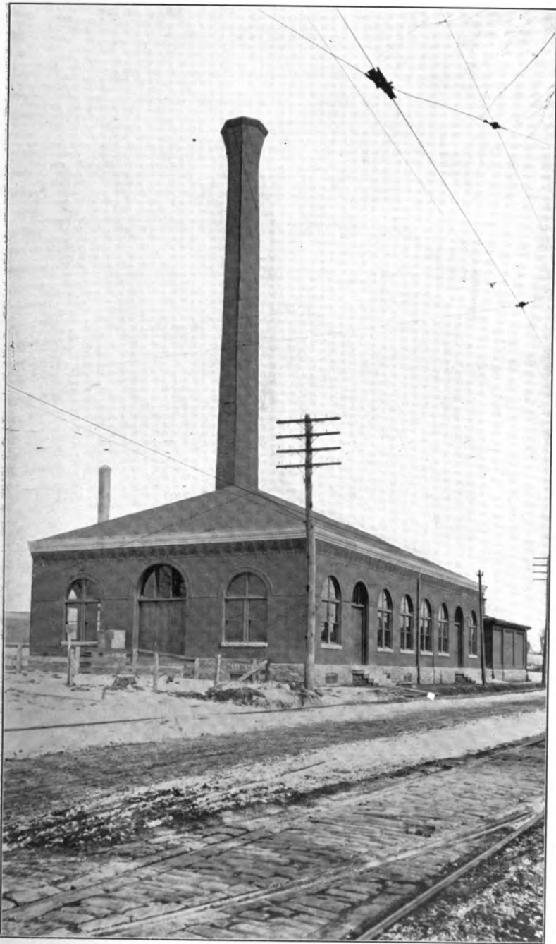
FRANKFORD HIGH SERVICE PUMPING STATION.
