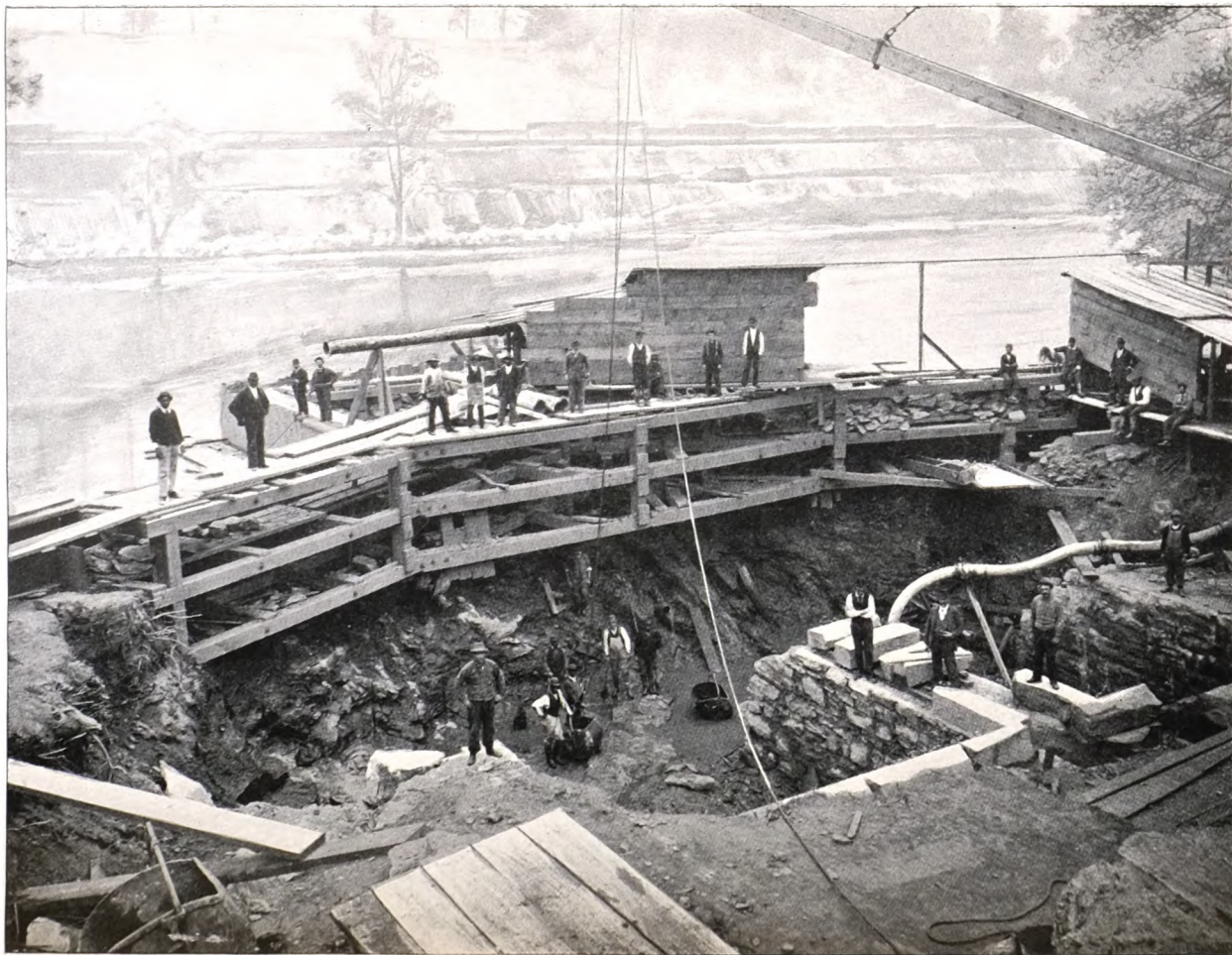
INTAKE UNDER CONSTRUCTION AT QUEEN LANE PUMPING STATION. VIEW OF DAM.
