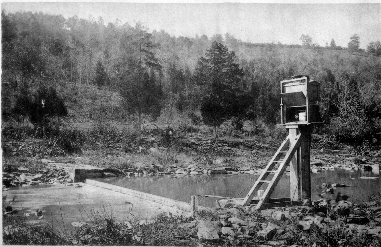
AUTOMATIC STREAM GAUGE AND GAUGING WEIR, Tohicken Creek, at Point Pleasant.
