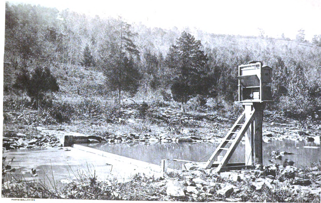
AUTOMATIC STREAM GAUGE AND GAUGING WEIR,
